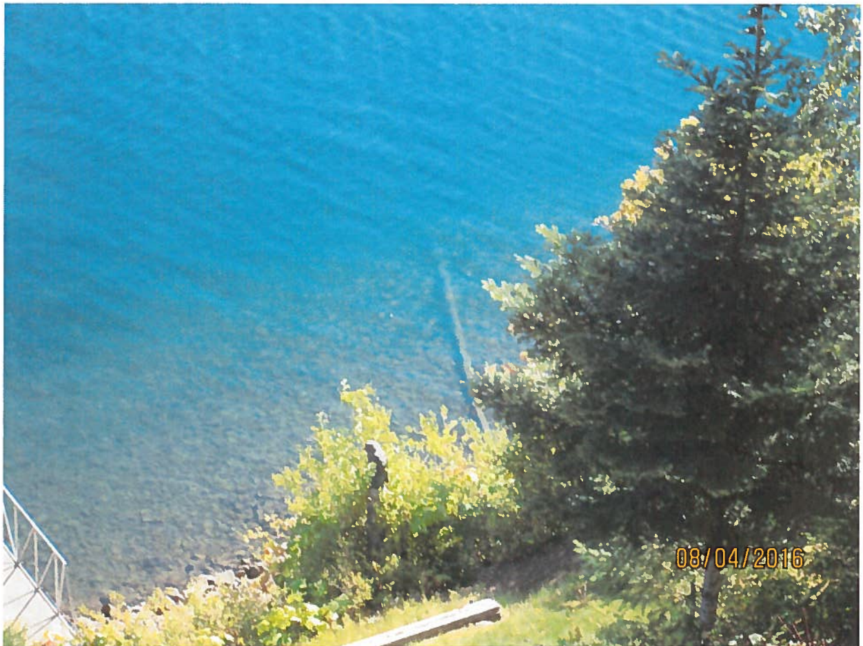
Pipeline from lake to shore.
