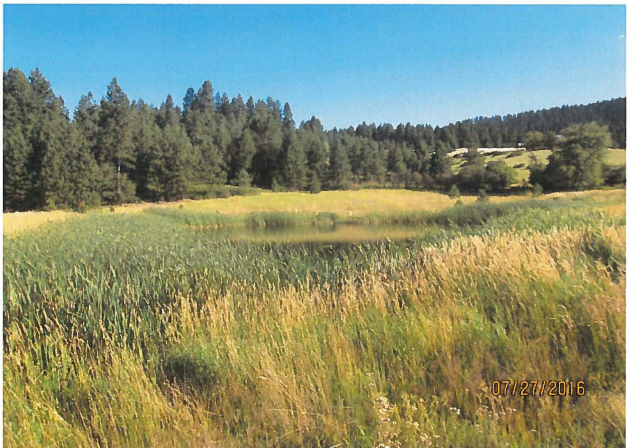
View of pond looking upstream from dam. Dam is located on left side of picture.
