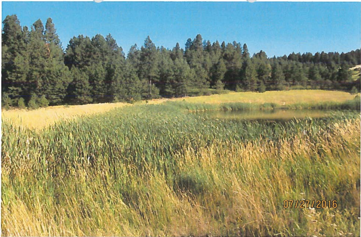
Dam is grassy area on left side. Overflow channel is below where cat tails are located.
