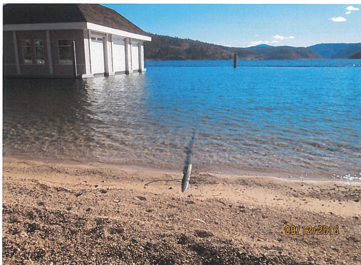
POD. 2 inch poly pipe.
