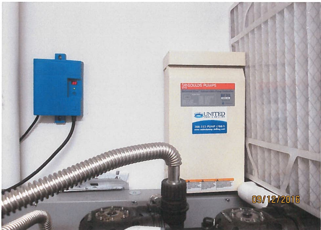
Verified system components with United Pump. 3 phase 3 hp pump set at 33 gpm.
