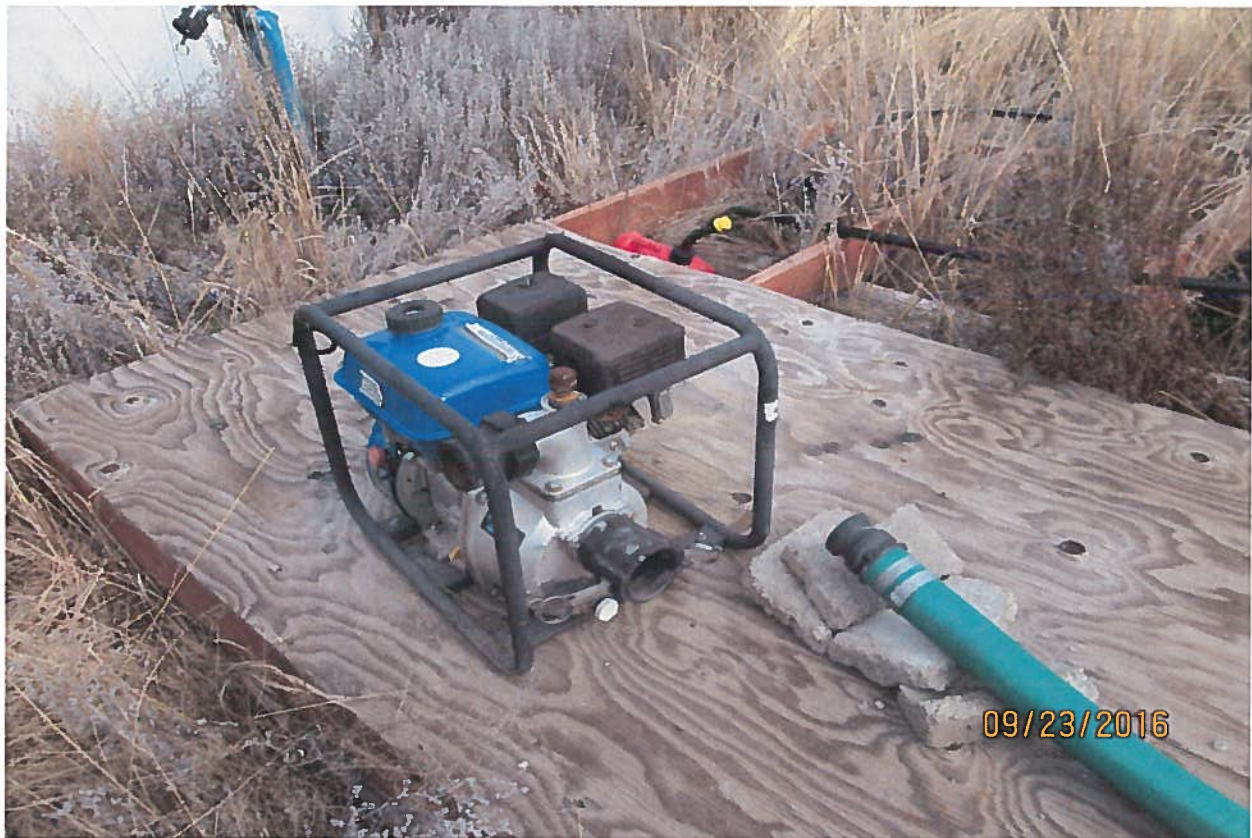
Small 1hp trash pump that was used to divert water from creek to cistern.
