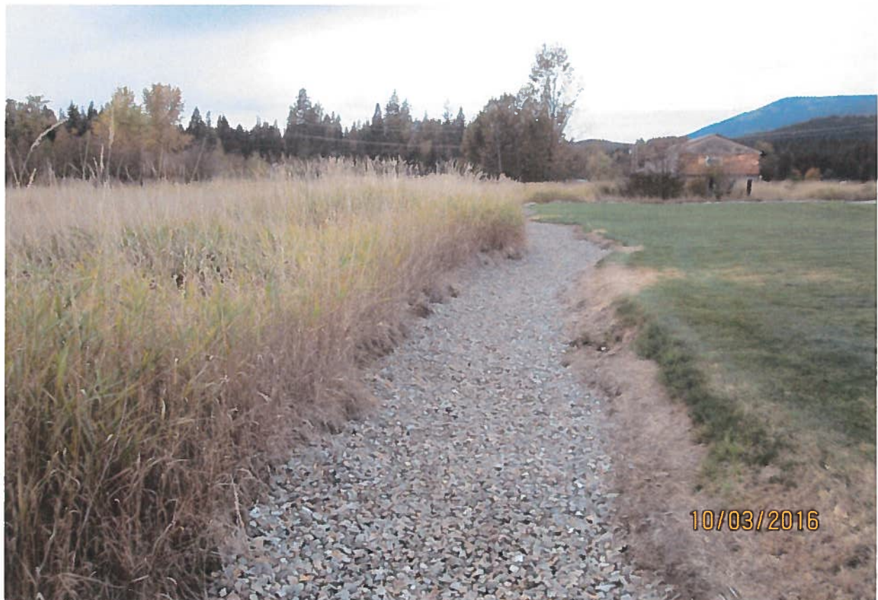
View from edge of pond looking west up unnamed stream.
