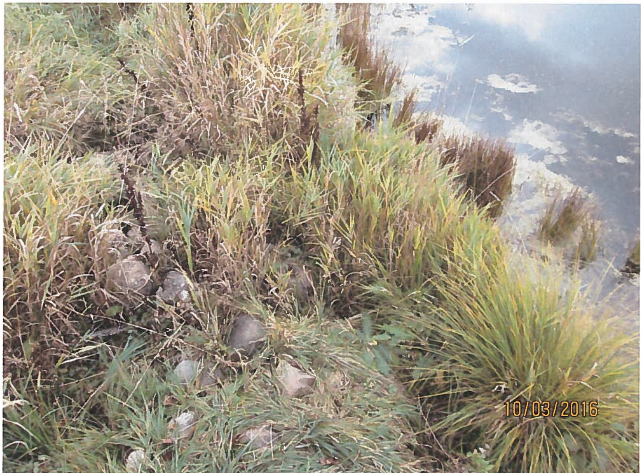
Dam on unnamed stream.
