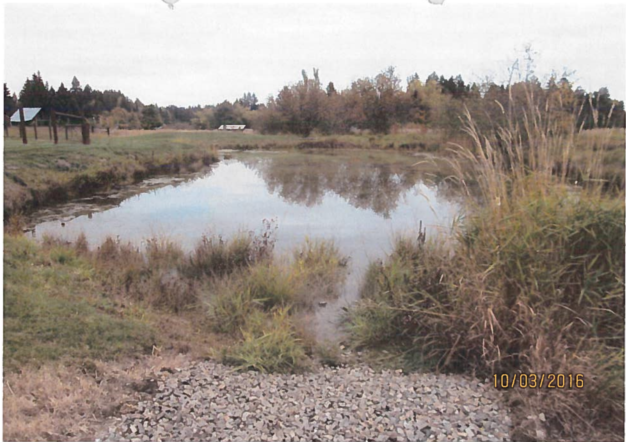
View looking west towards dam from unnamed stream which was dry and seasonal.
