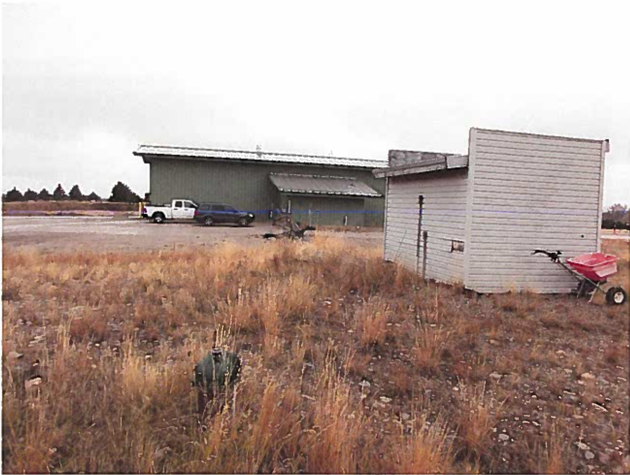
Looking west at pump house in the foreground and scale house in background.
