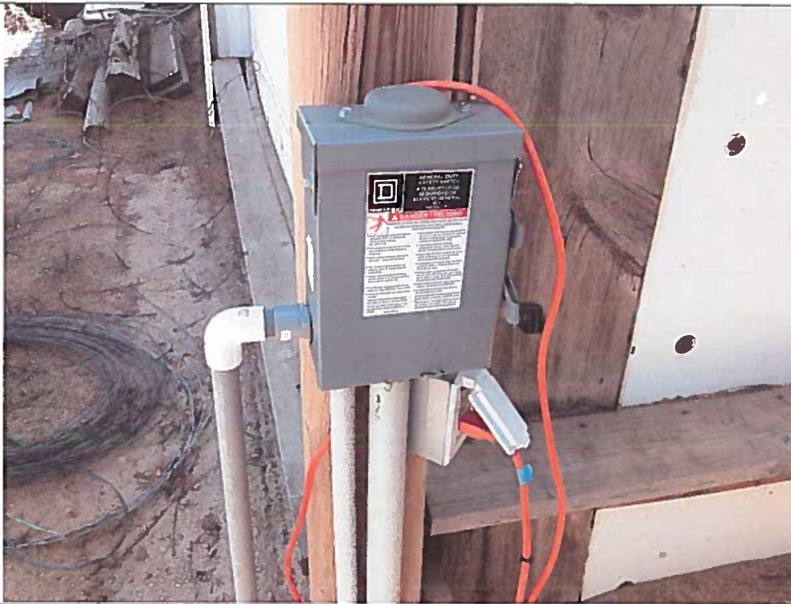
Power source with lockable control.
