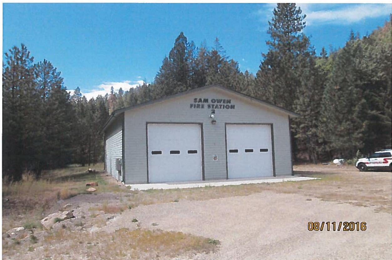
Fire station and some light irrigation around to keep fire danger lower.
