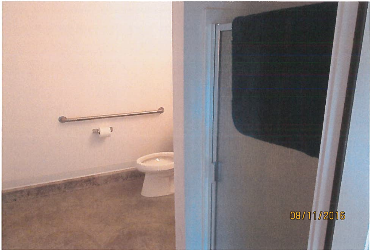
Bathroom in fire station.
