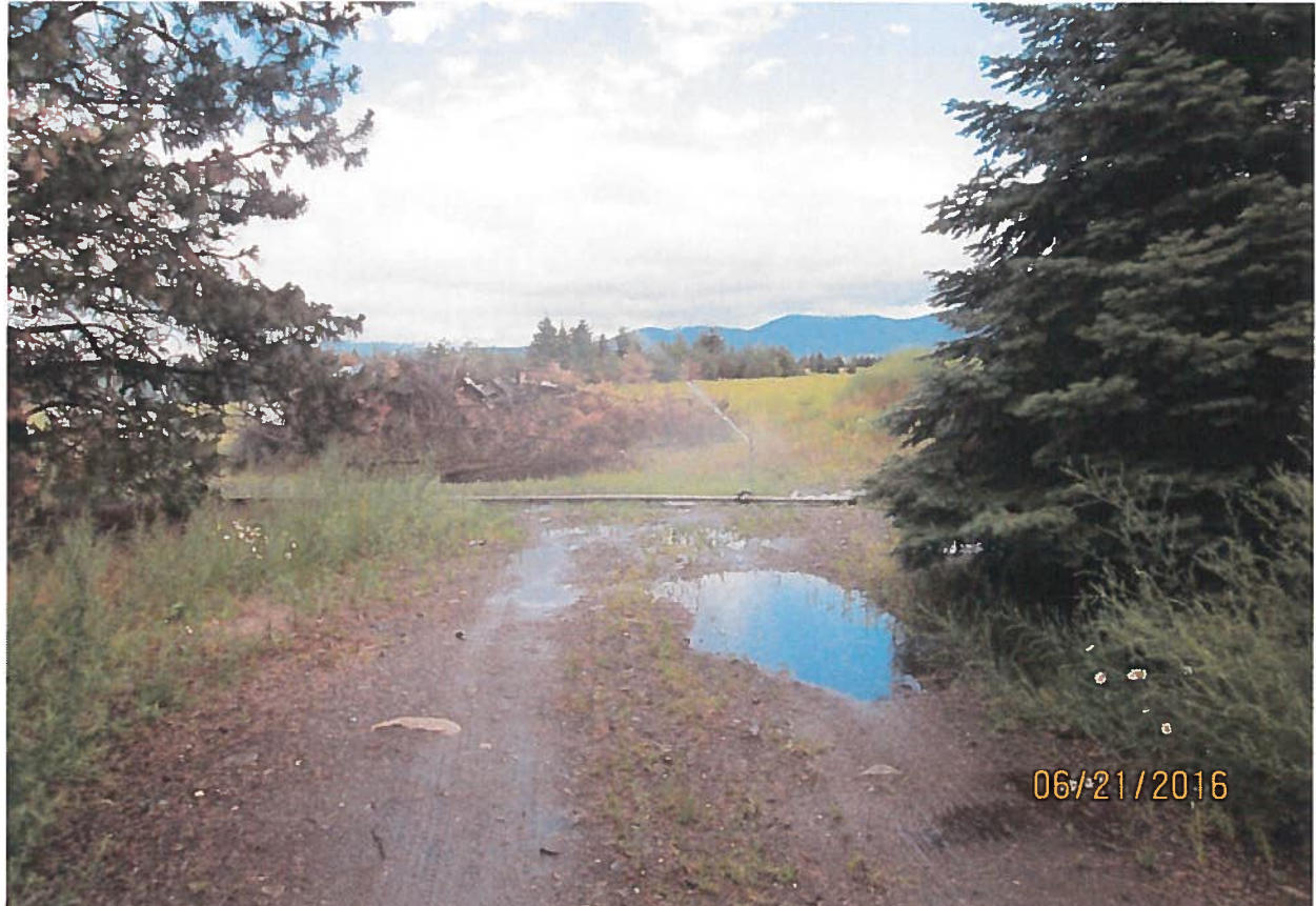
3 inch aluminum pipe with rain bird 5/32" heads. Running at 60 psi each head can produce 5.47 gpm.
