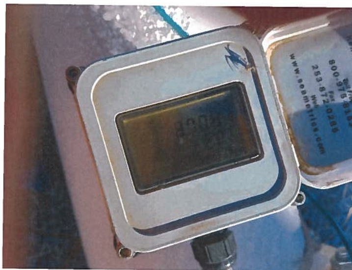
Figure 5. Well No. 2 flow meter – November 29, 2016 (totalized volume in acre feet)
