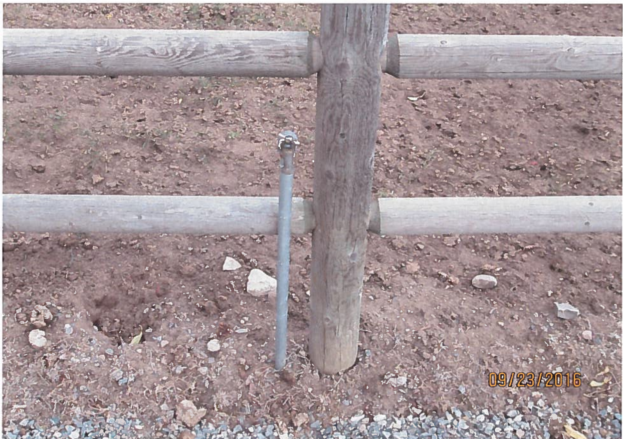
Frost free hydrant for use for irrigation or stockwater filling.
