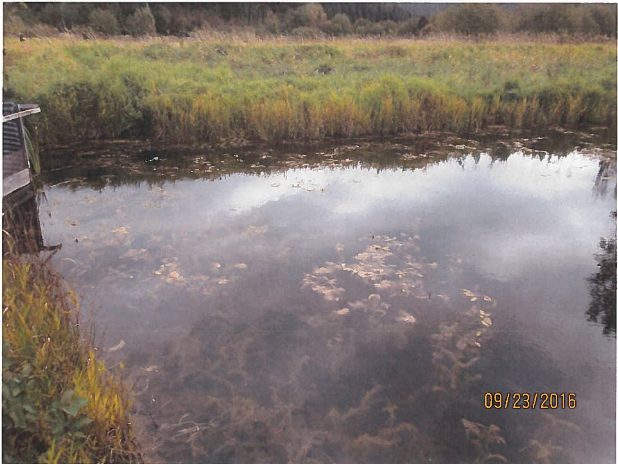
Standing on dam with discharge culvert for pond.
