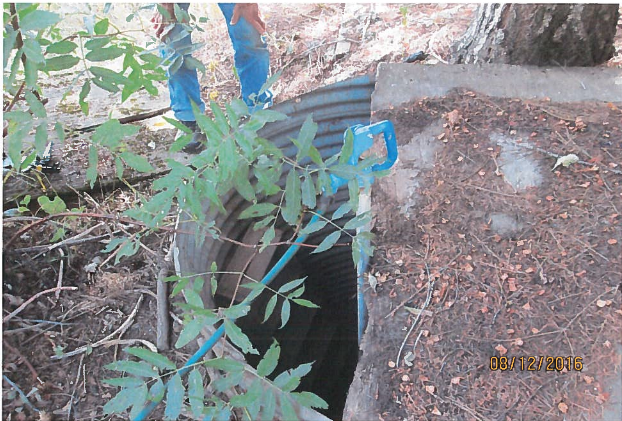
Frost free hydrant coming from well. 5 gallon bucket test performed showing 12 gpm.
