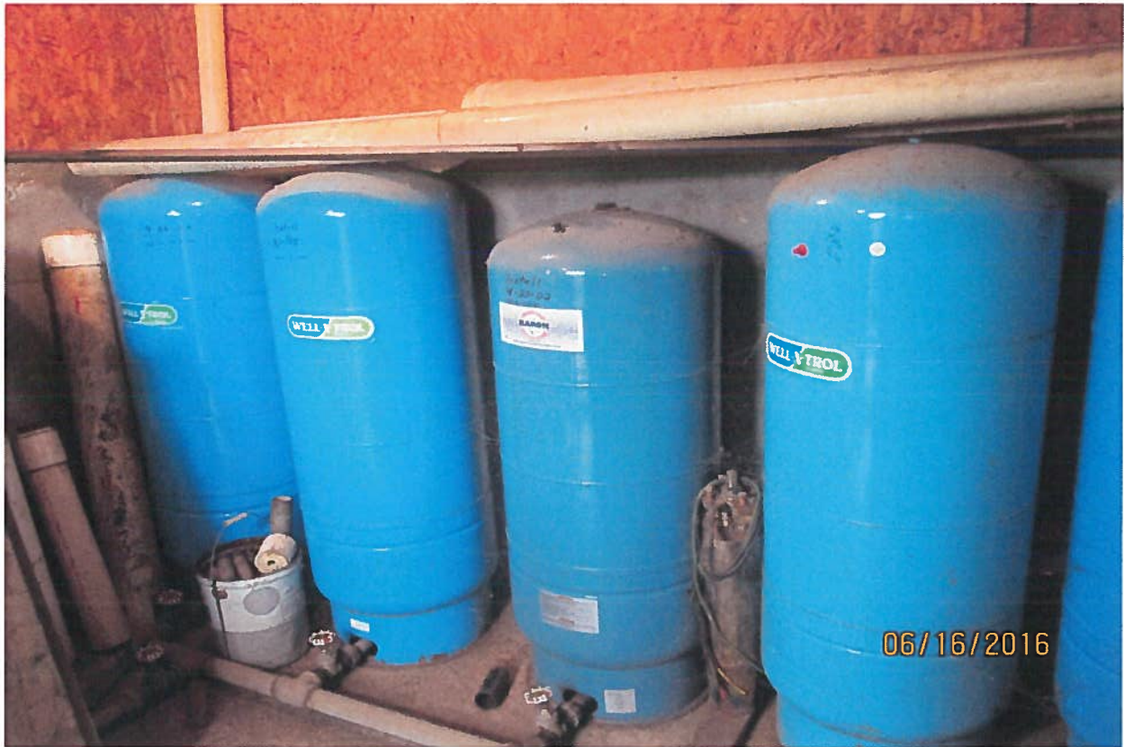
Individual home pressure tanks adjacent to well.
