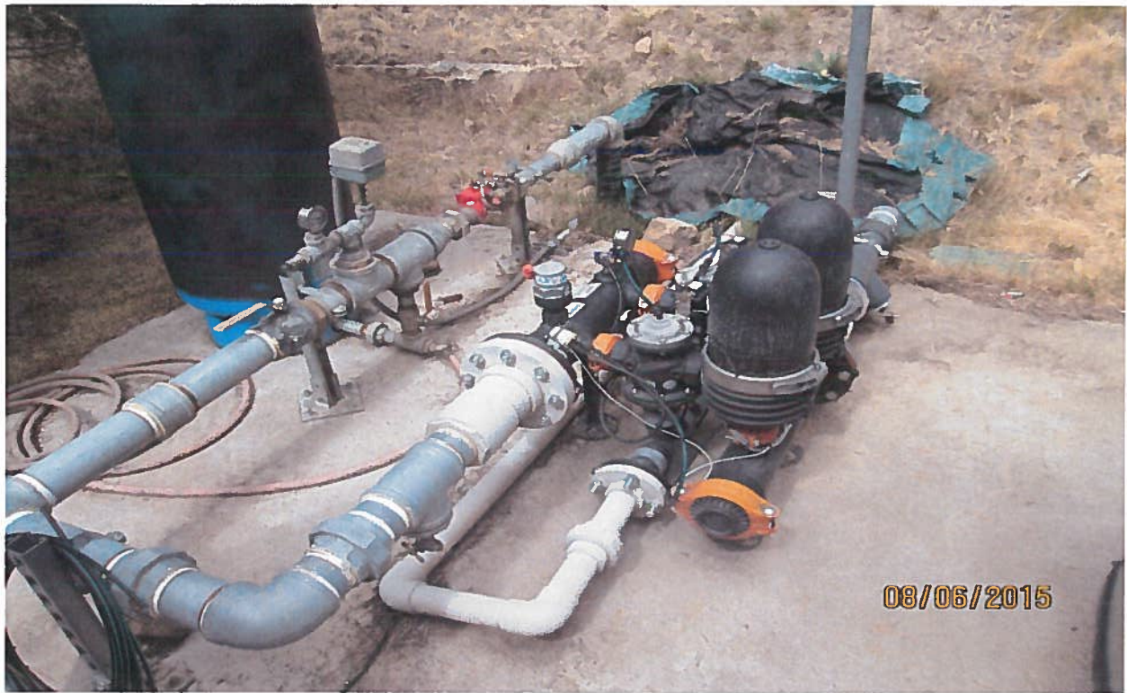
Filtration system for lake water. Water is pumped from lake to filtration to small storage tank and then pumped to irrigation system.
