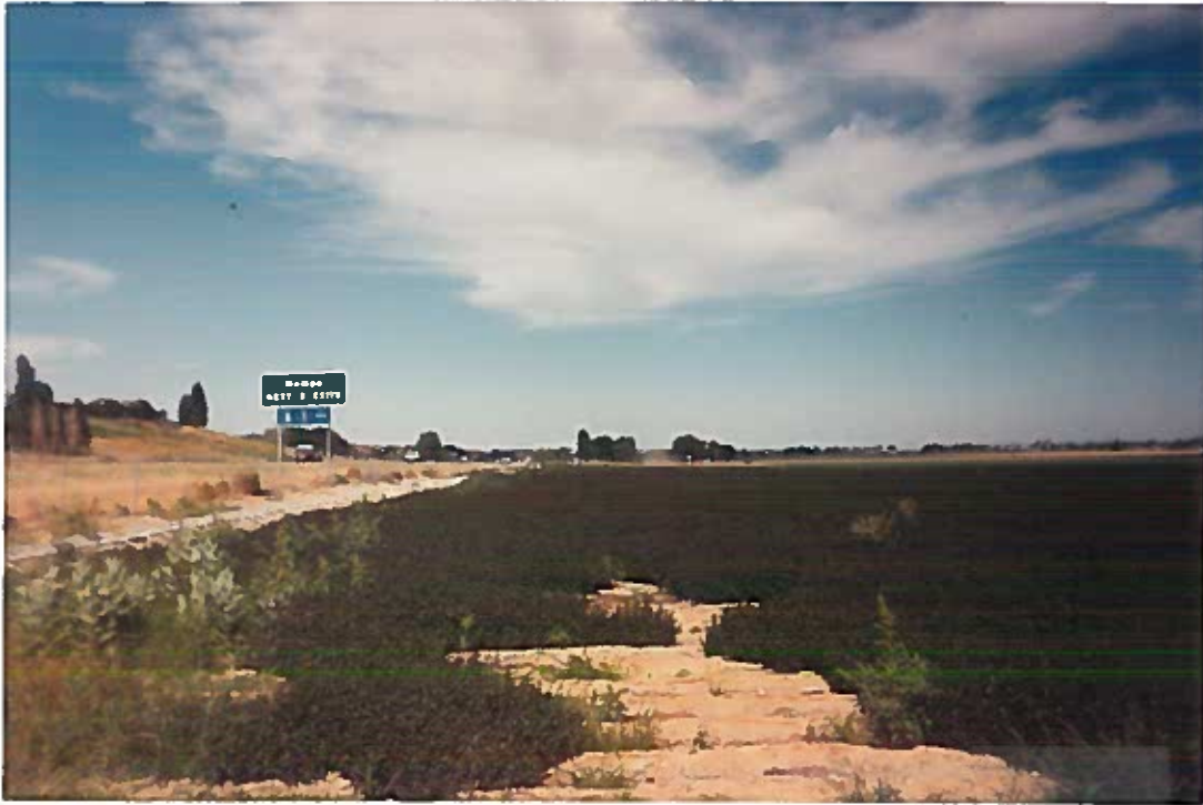
View of the mint field : concrete ditch system
