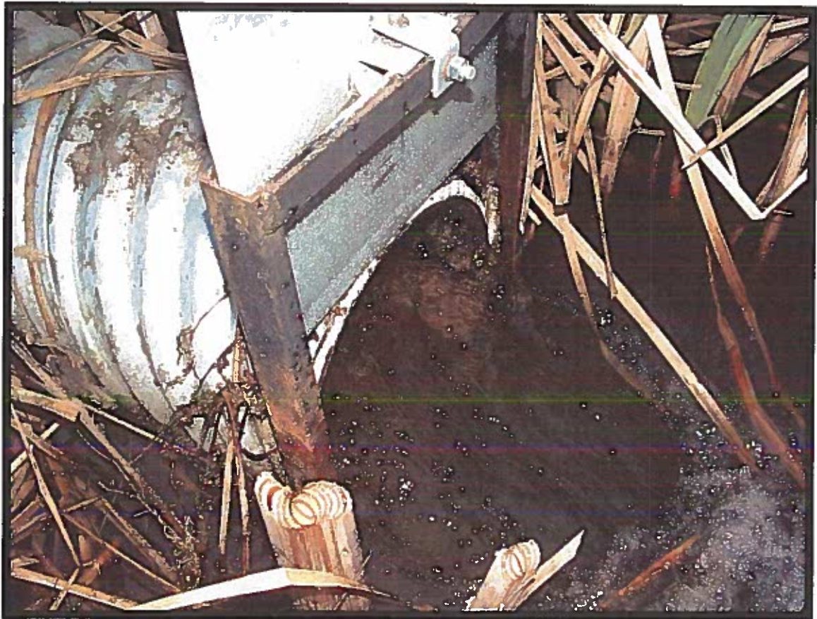
Diversion Works: 12-inch Corrugated Pipe
