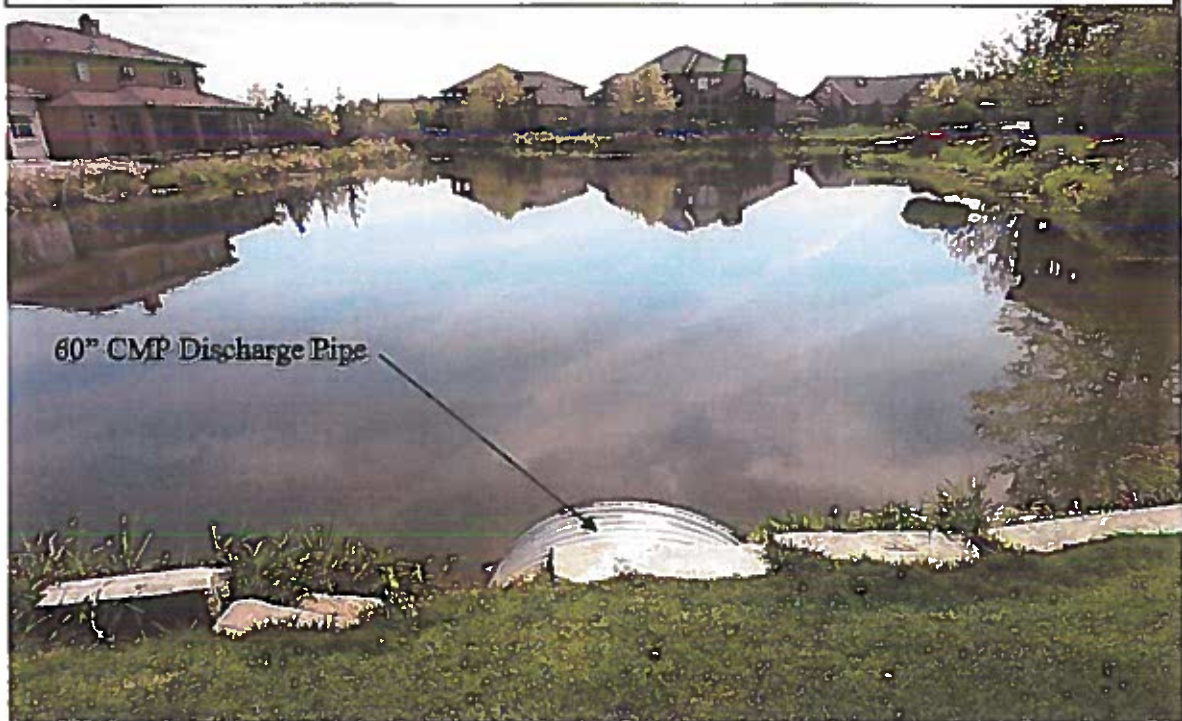
Place of Use: View southeasterly of the HOA aesthetic storage pond within the Banbury Meadows development. The 60" CMP discharge pipe is located at the west end of the aesthetic storage pond.
