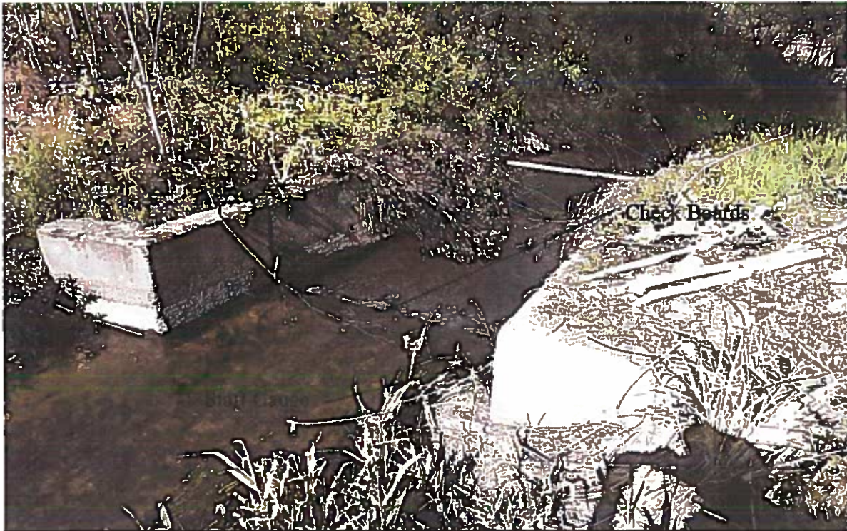
View southwesterly of a concrete flow measuring structure in Warm Springs Creek. The structure is approximately 100' downstream from the 36" CMP discharge pipe from the Boise River. A staff gauge is mounted to the northerly abutment upstream of the flow control boards.
