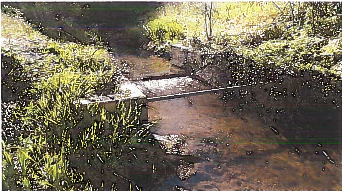
View southeasterly and upstream of the headwaters of Warm Springs Creek and the concrete flow measuring structure.
