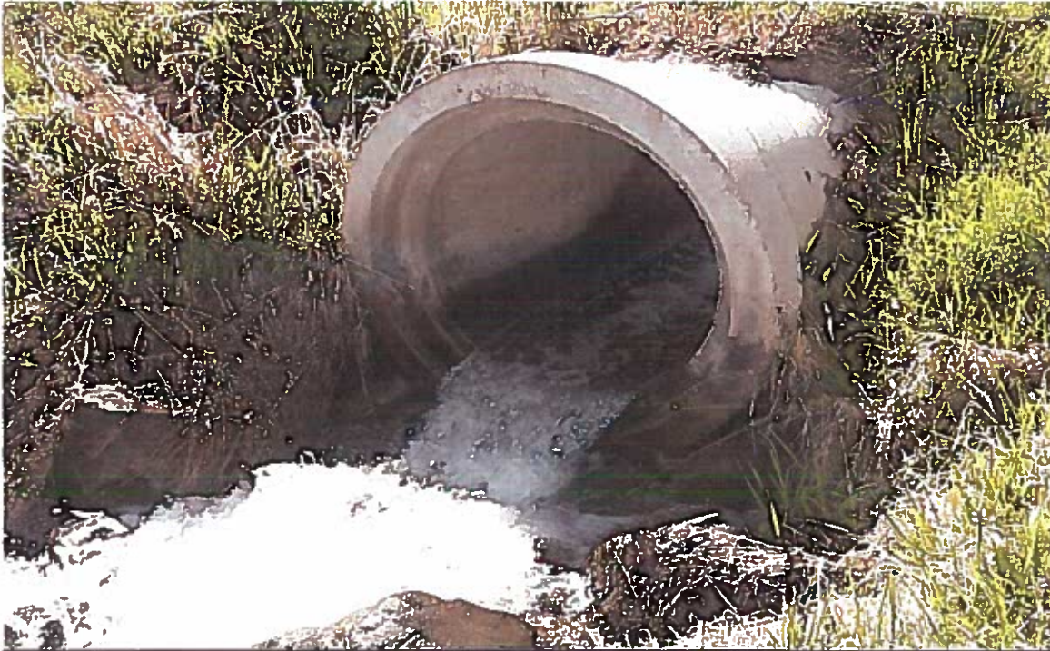
View southeasterly of the 48" RCP pipe discharging water from the concrete irrigation structure serving the property owner's adjacent to Eagle Road back to Warm Springs Creek.
