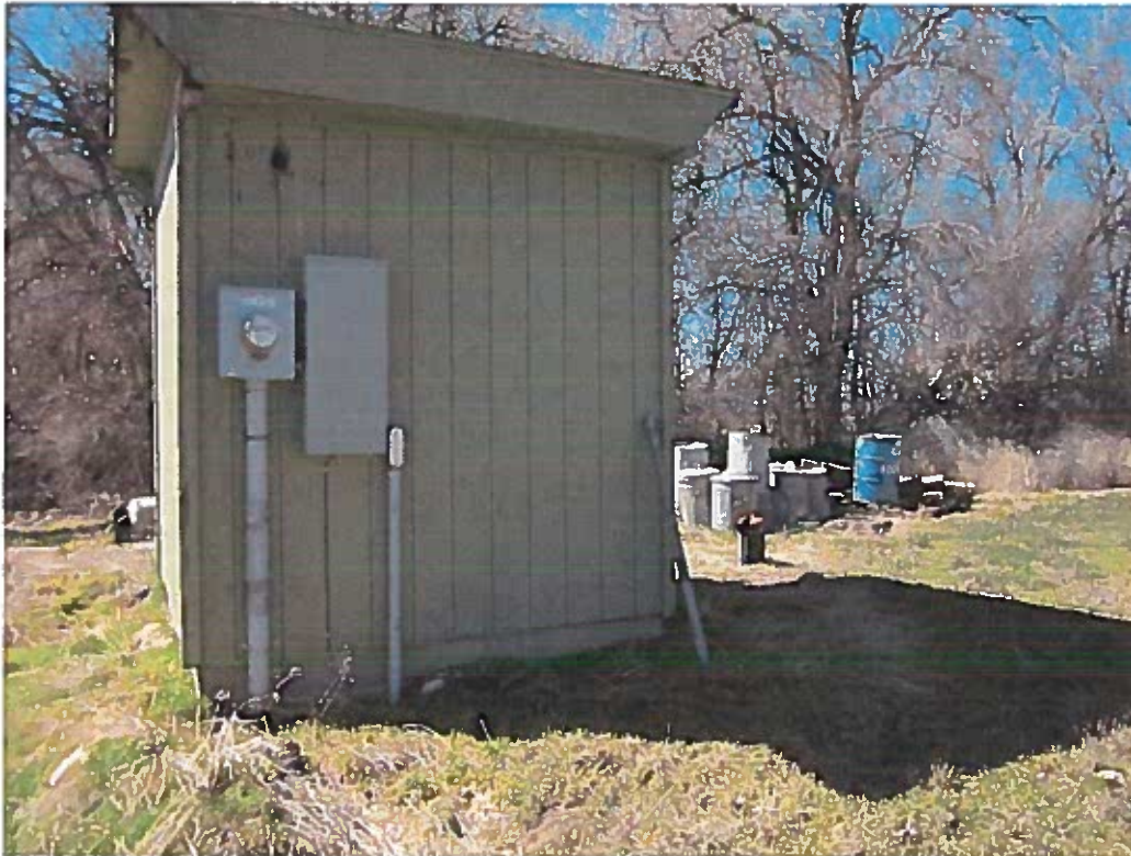
Figure 3: Pump house and well.
