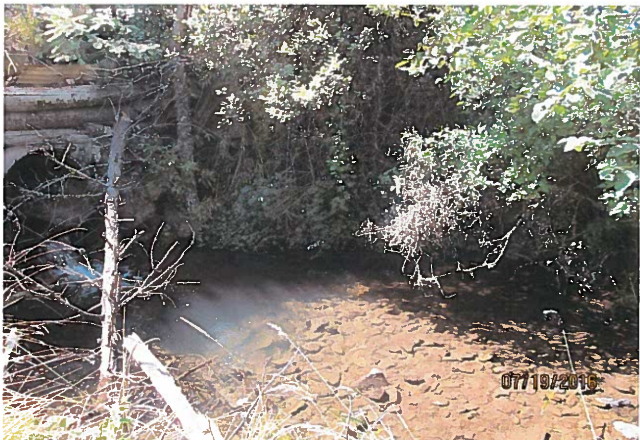
Point of diversion on unnamed stream in Lot 2. Pump would go down in pool area next to culvert.
