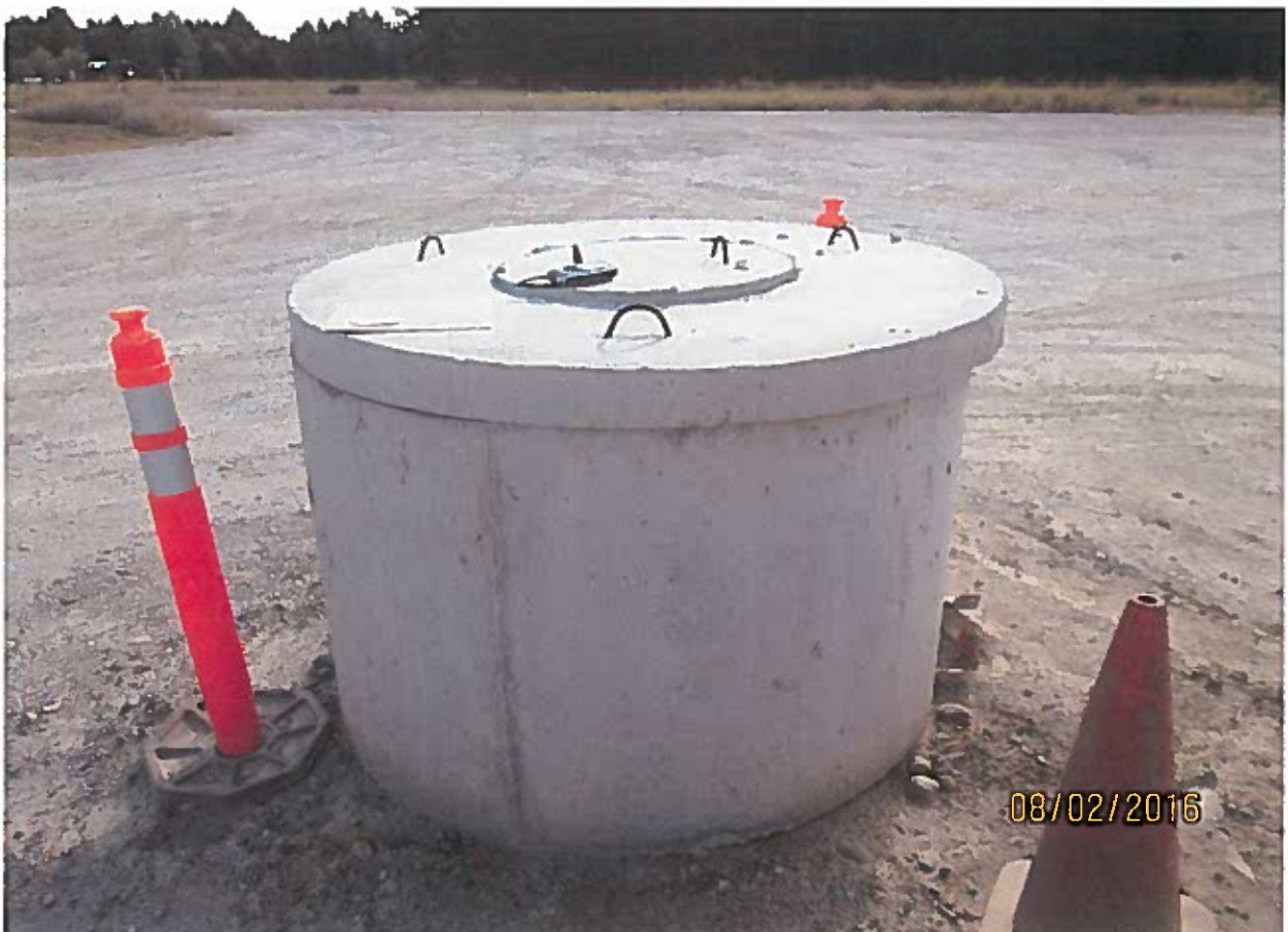
Well location. Could not access because of concrete cistern to protect location from trucks. Given IDWR tag A0020003.
