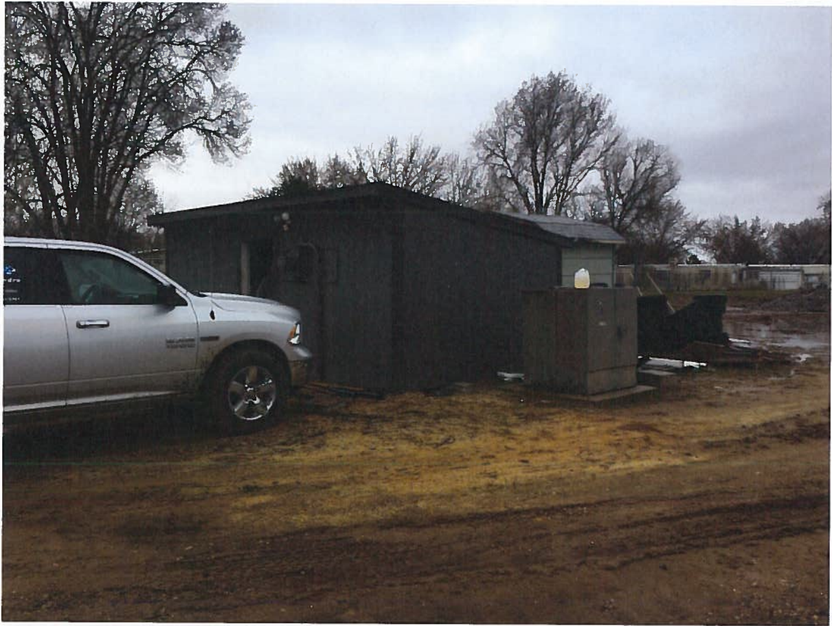
1. Well house building exterior
