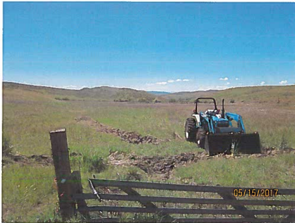
Figure 1 Looking south from the excavated diversion ditch towards the irrigation place of use.
