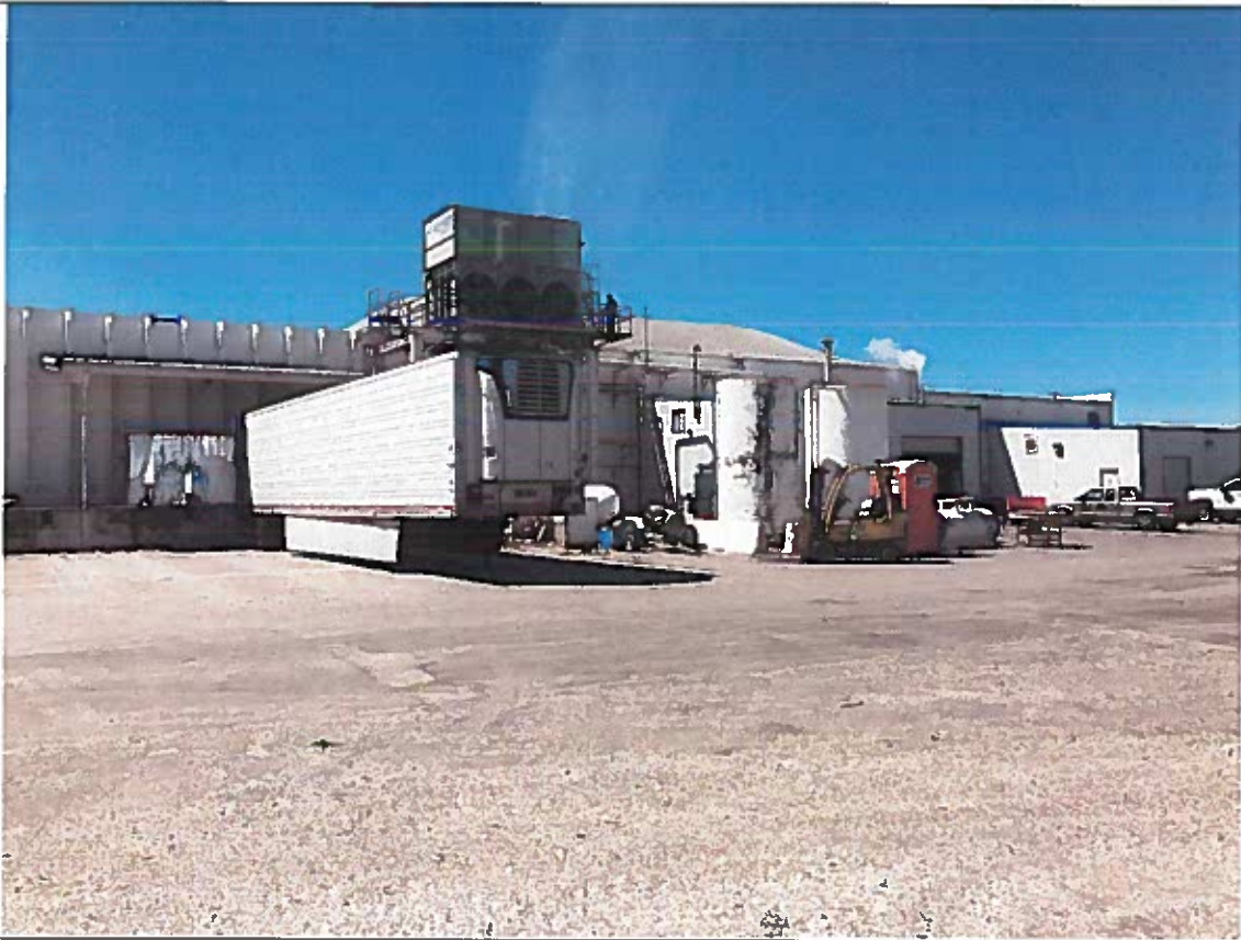
Onion processing plant. (POU)
