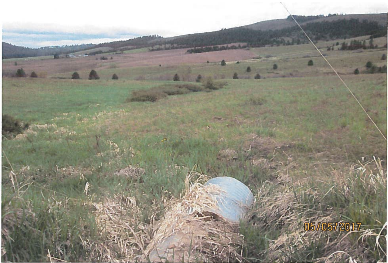
View down draw from culvert from pond.
