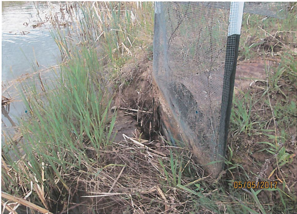
Protected culvert for overflow in pond.
