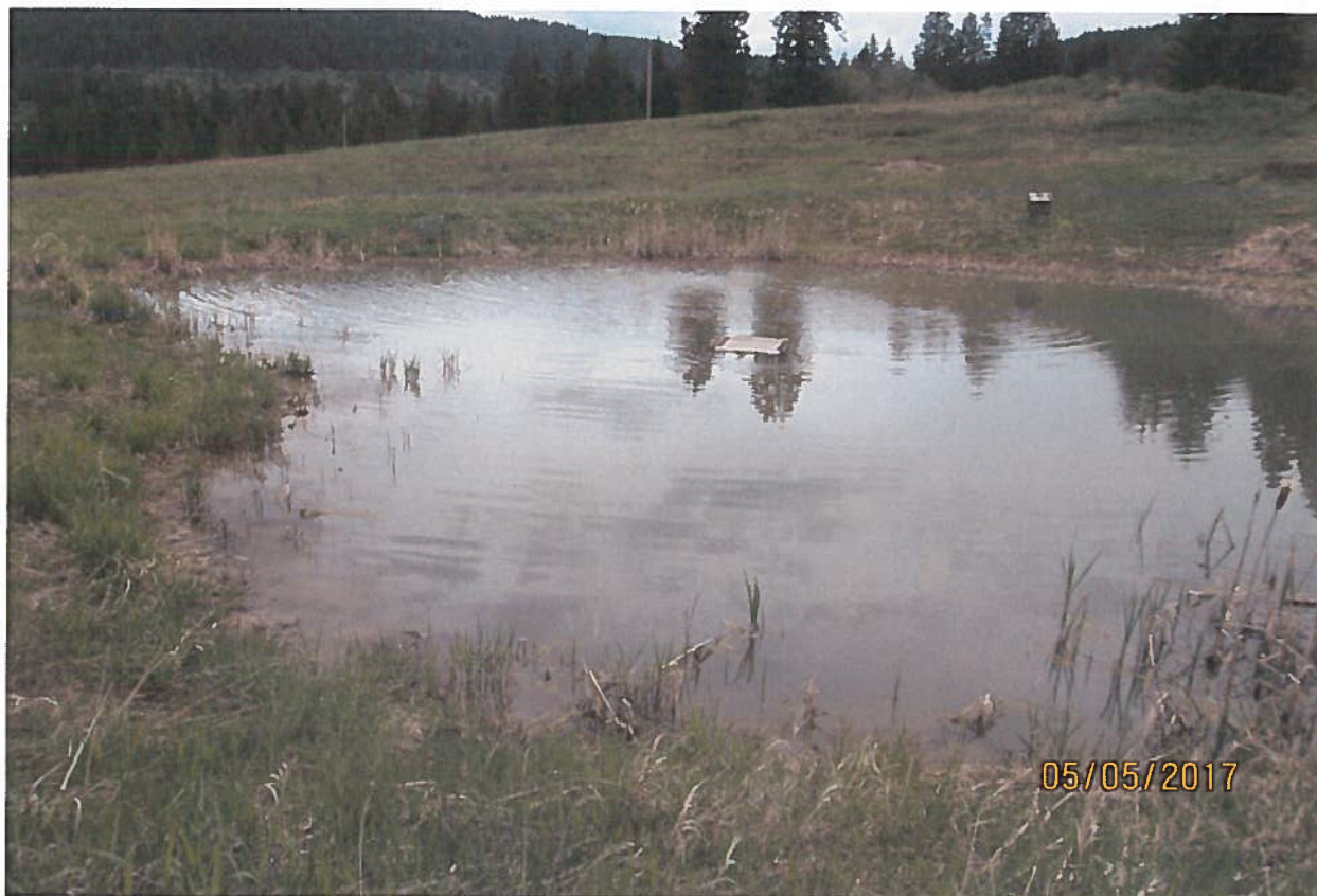
View looking at outlet culvert and dam.
