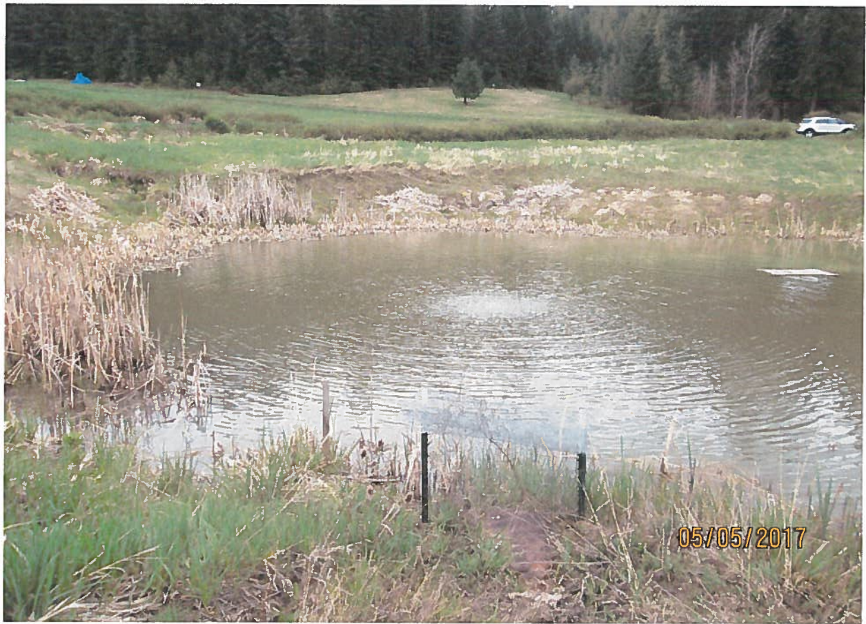
View from culvert towards pond.
