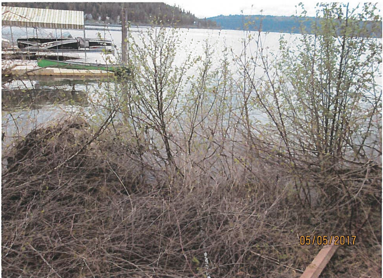
View of pipe in bottom going into lake.
