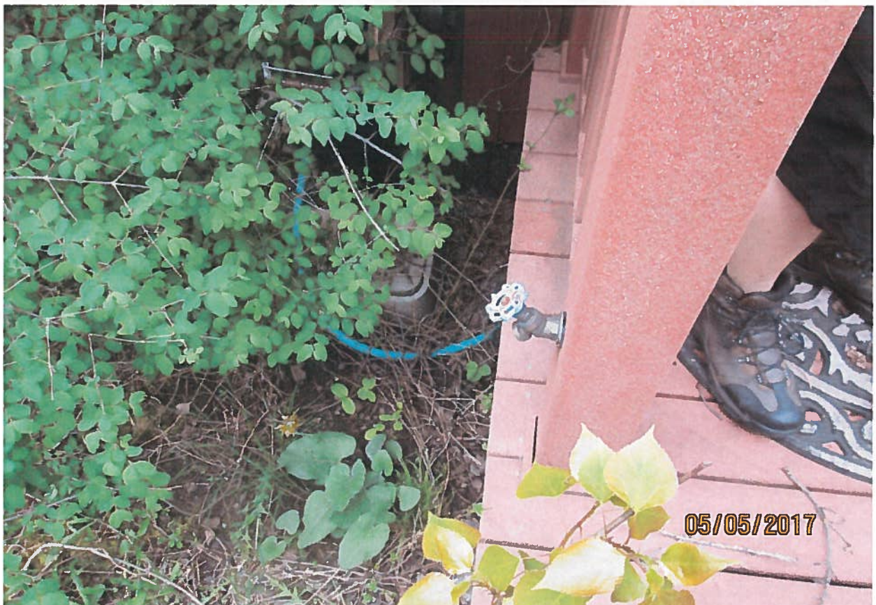
1 of 3 faucets that was fed by lake water. Small quarter inch line was plumbed under deck to hose nozzles.
