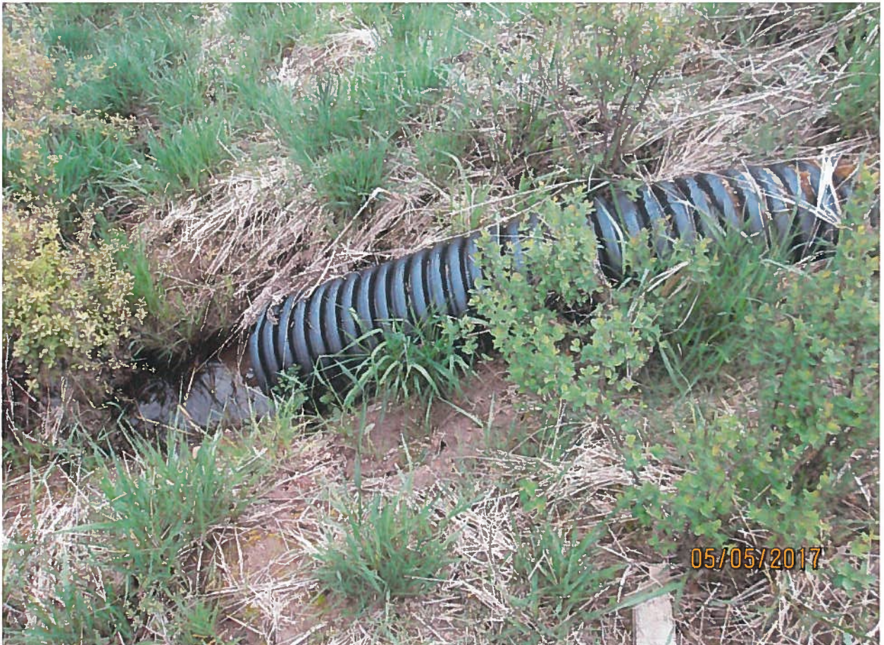
View of outflow culvert.
