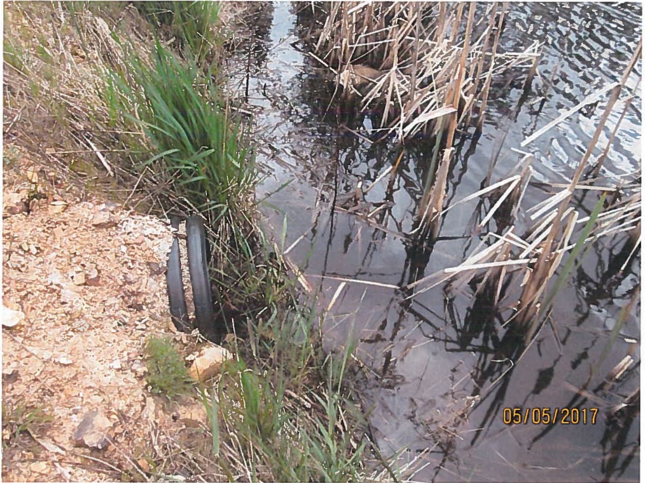
Overflow culvert in dam.
