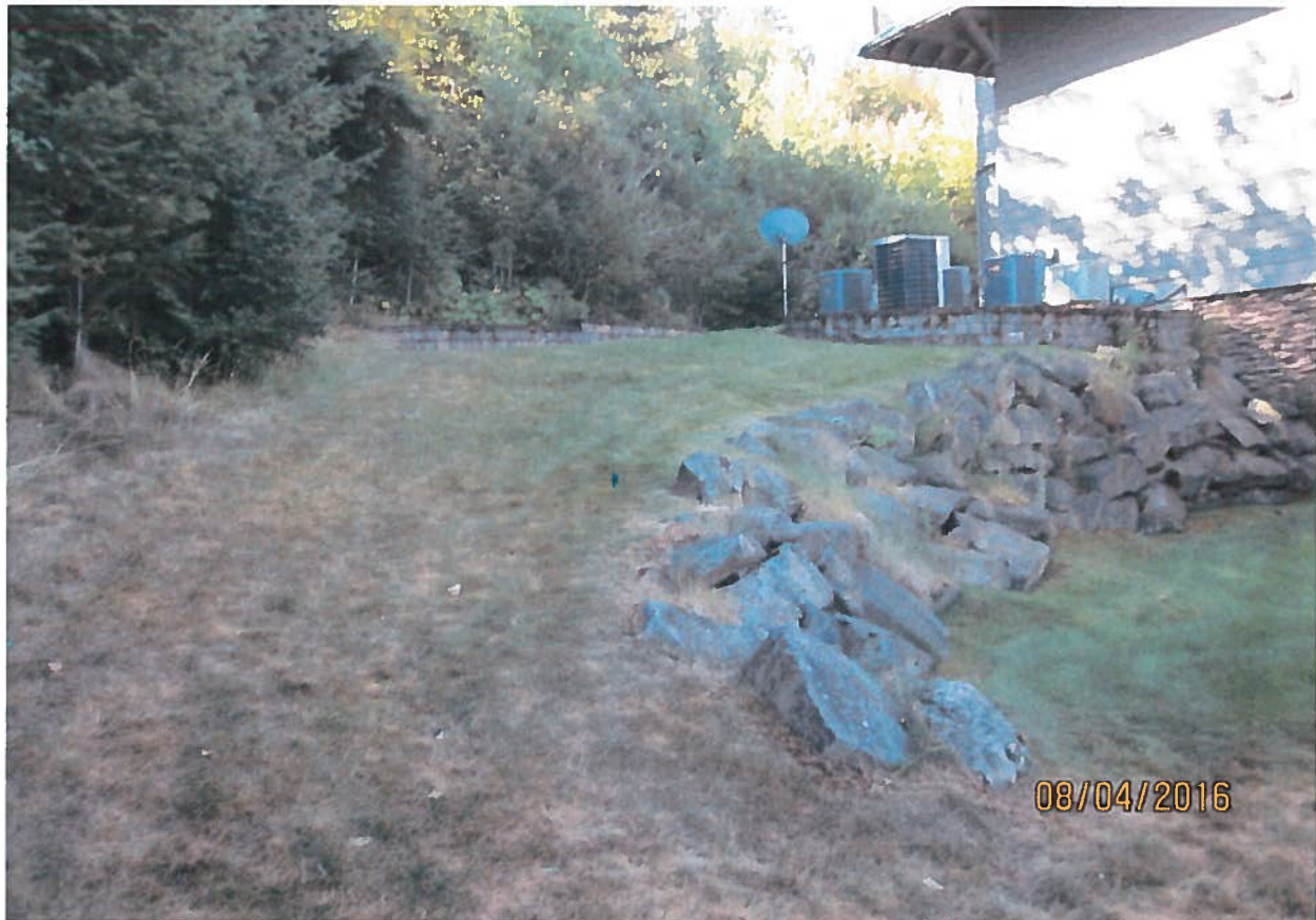
Irrigation and area where pipe from lake goes up hill to storage tank.
