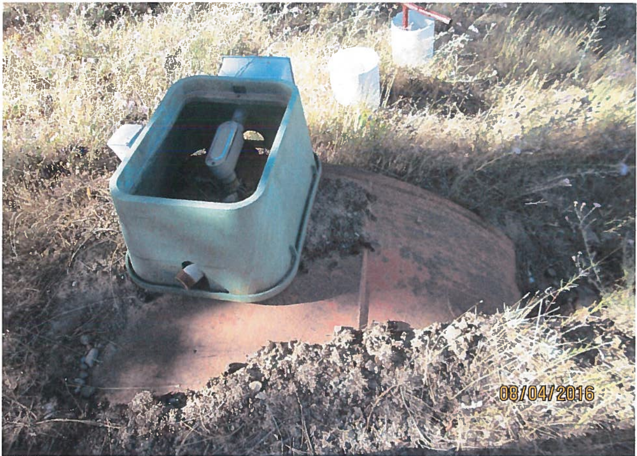
Electrical box on edge of storage tank for irrigation from the tank.
