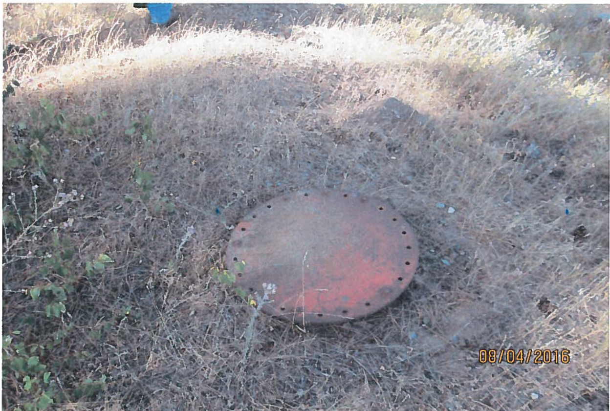
Top of storage tank.
