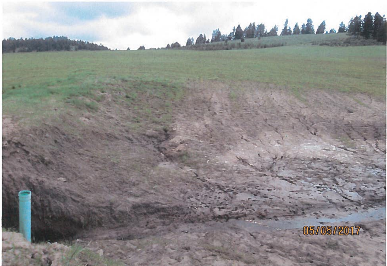
View from dam at overflow culvert and storage area.
