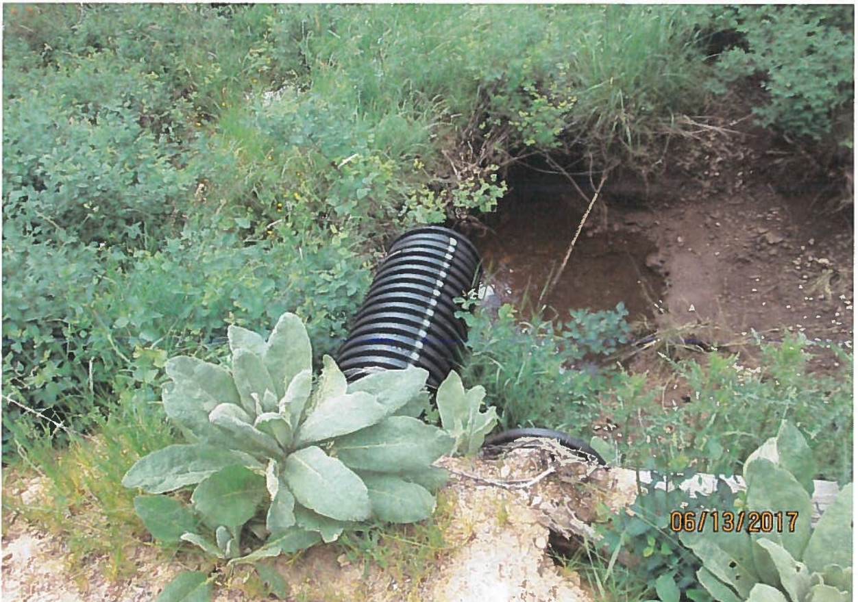
Overflow culverts looking downstream from dam.
