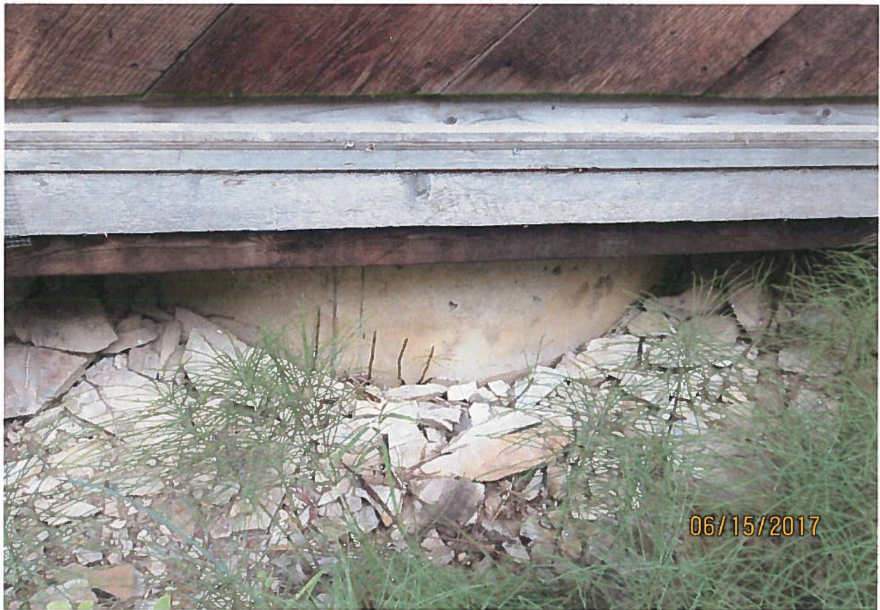
Concrete ring under well house.
