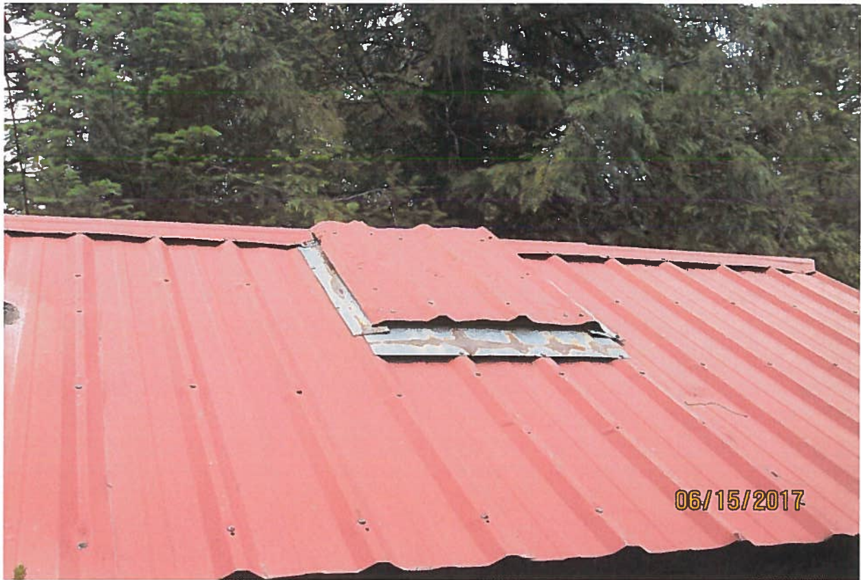
Access whole in roof for pump replacement.
