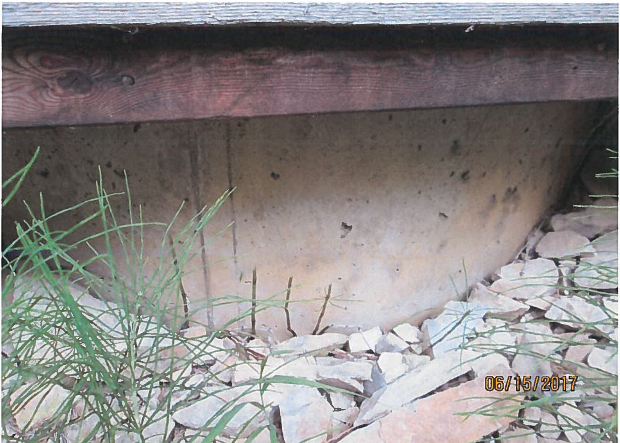
Concrete ring used for hand dug well.
