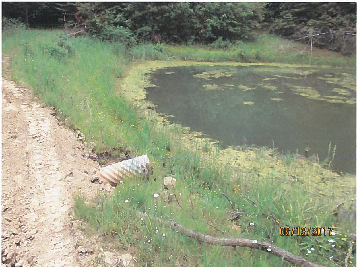
Dam with overflow culvert.
