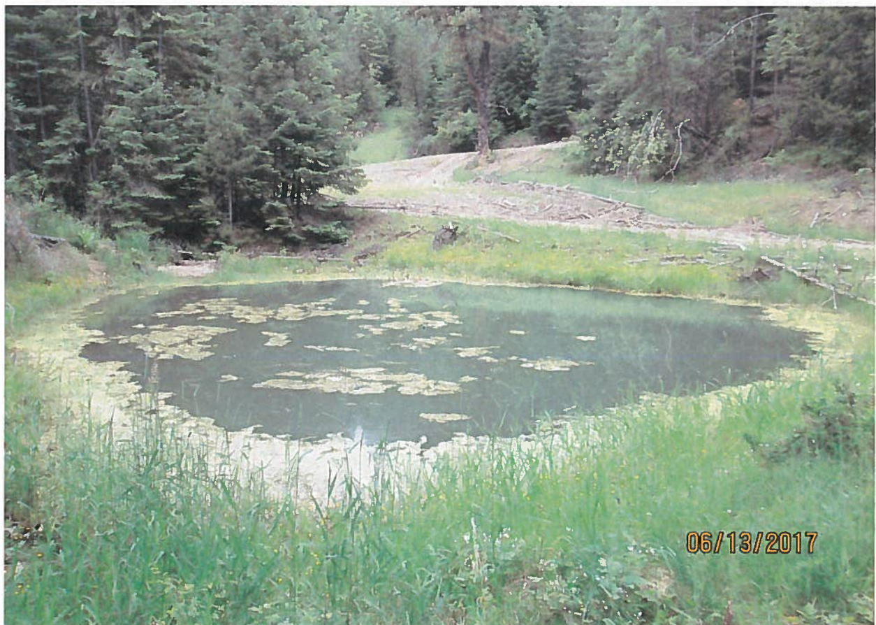
View of pond from dam.
