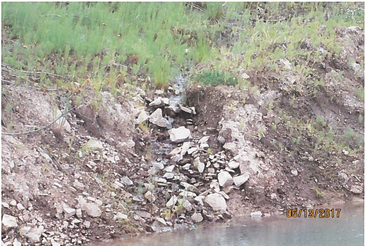
Water flowing in from unnamed stream.
