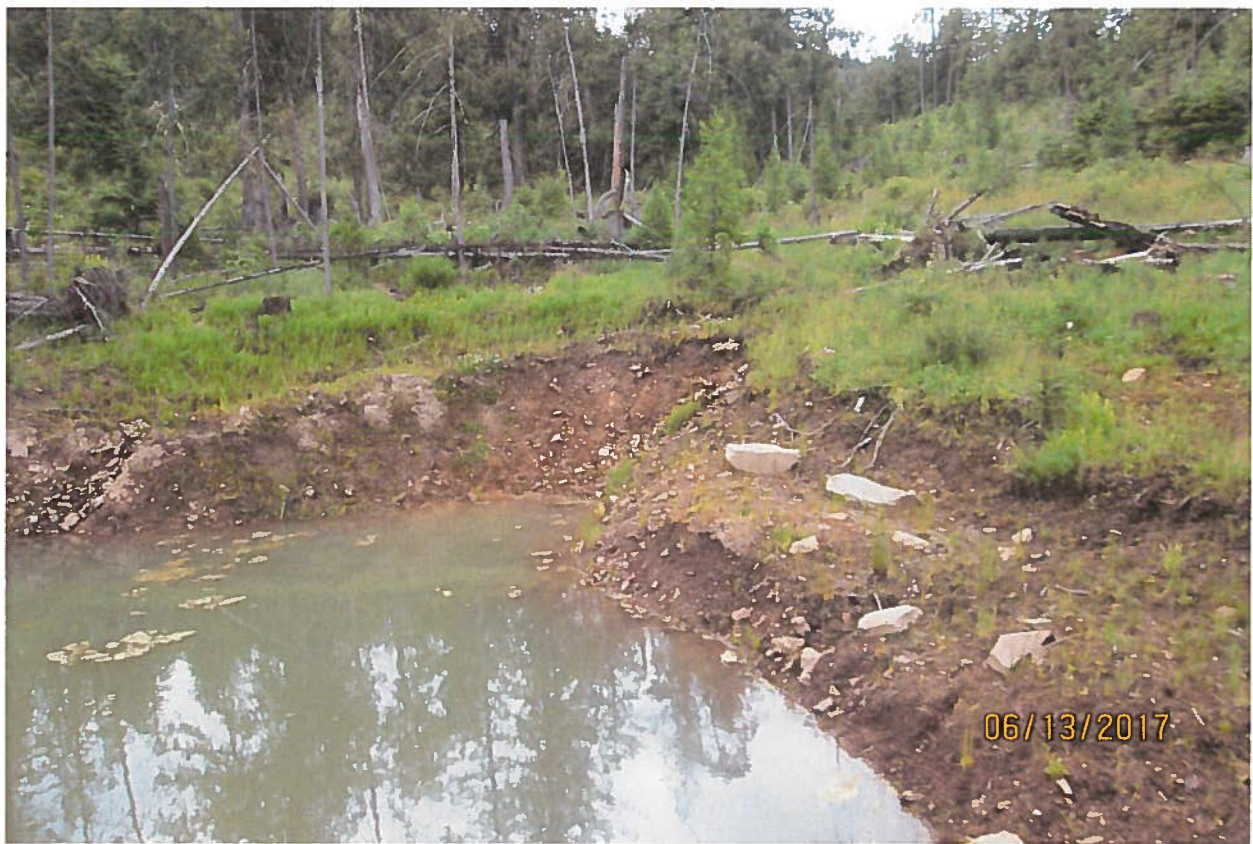
View of pond looking uphill at drainage area.
