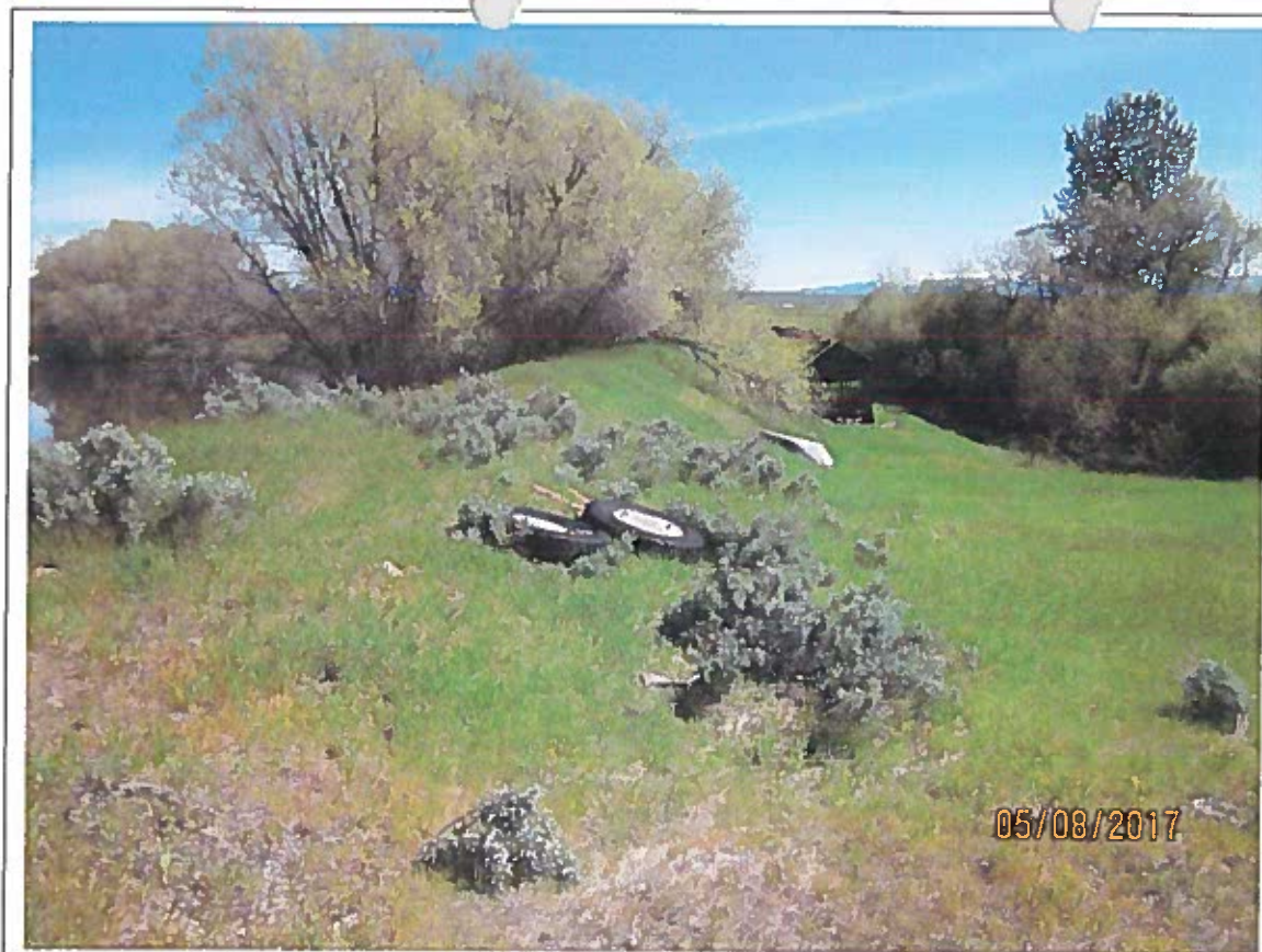
Toe of dam looking northeast.
