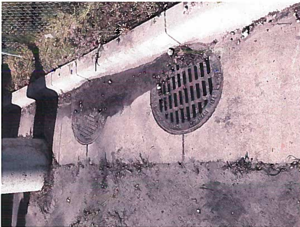
Precipitation drains to storm drain system.
