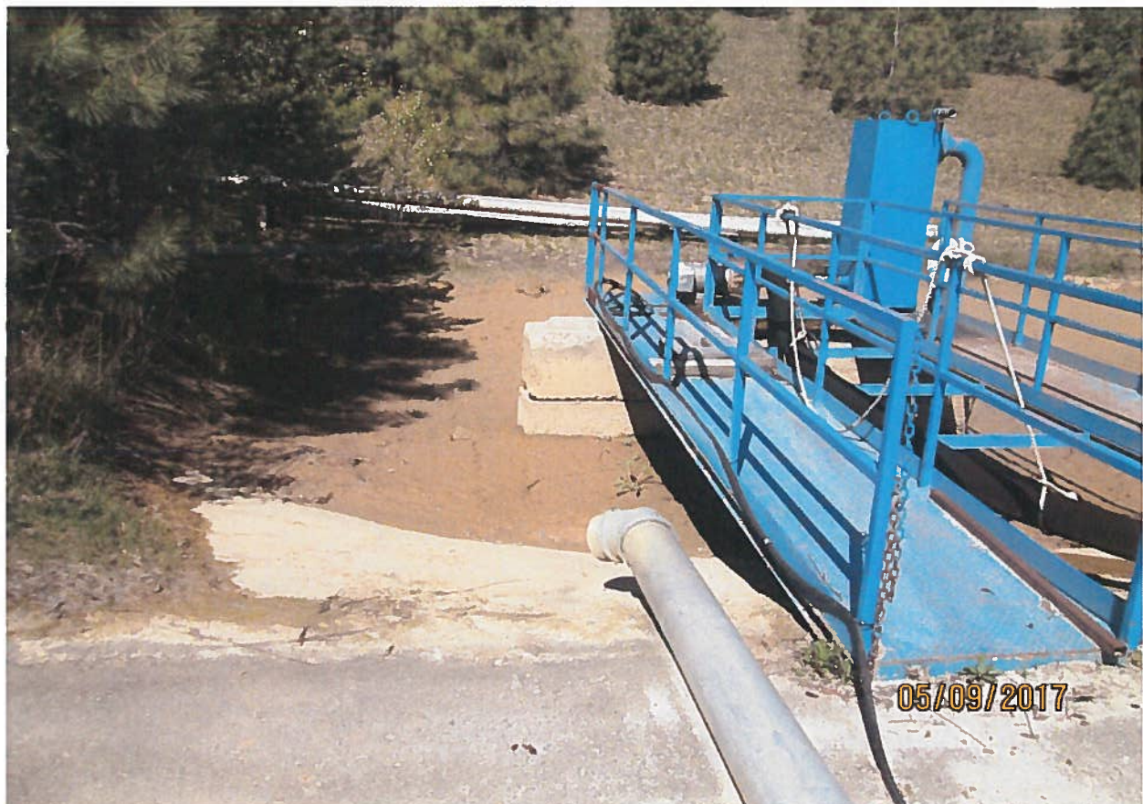
Asphalt lined settling pond.
