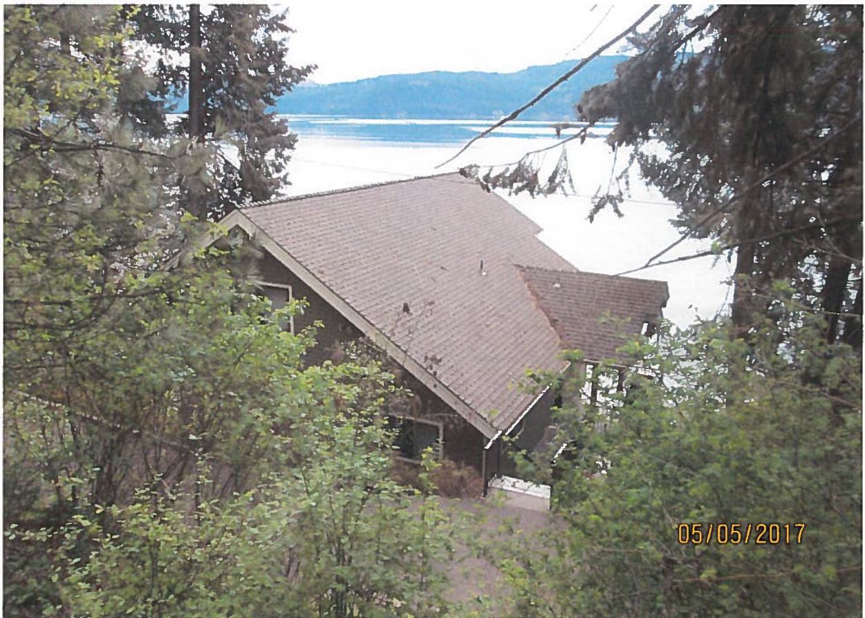
Home 5 served domestic water and irrigation.
