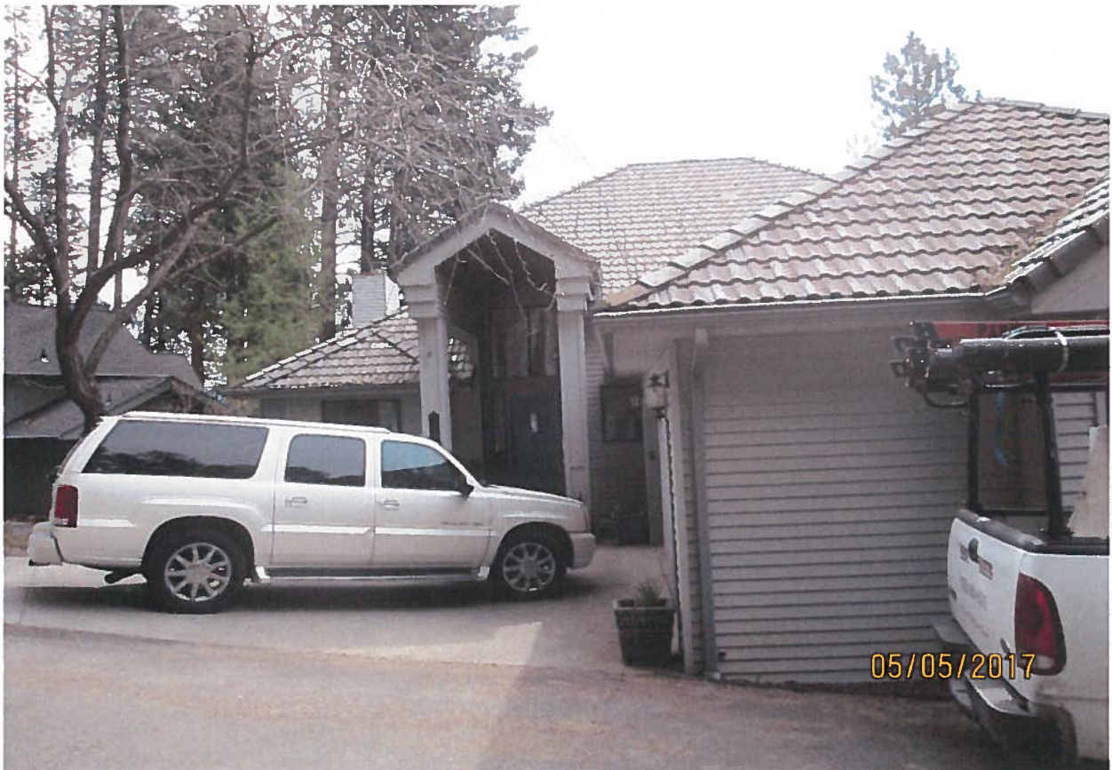
Home 11 served domestic water only.
