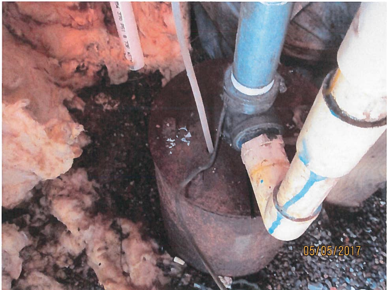
Well serving homes that was drilled in 1984 to a depth of 180 feet. Given IDWR tag A0020018. SCANNED JUN 14 2017
