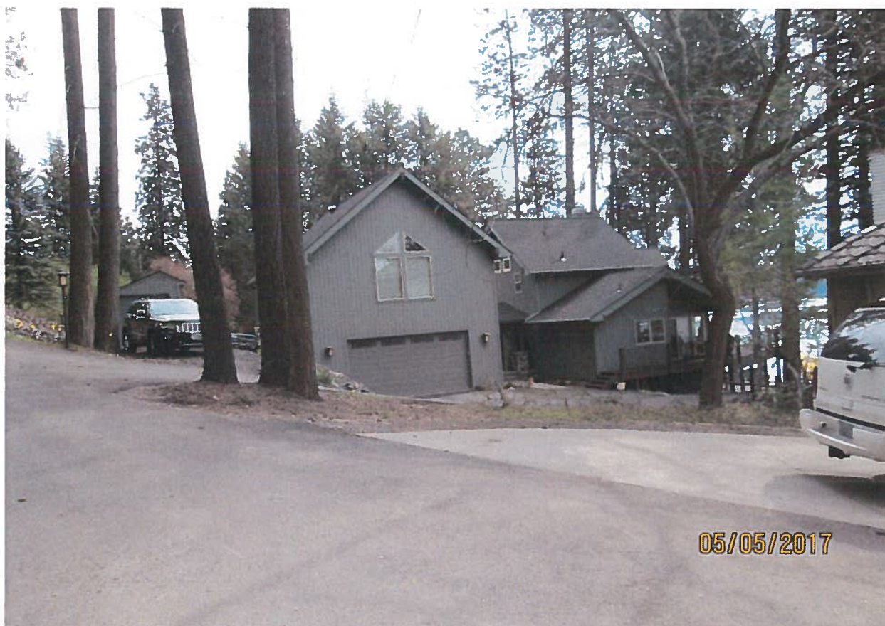
Home 12 served domestic water only.
