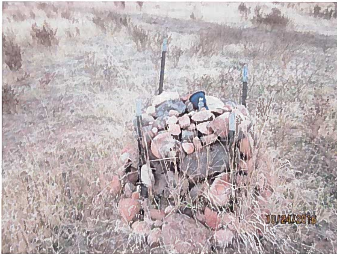
One of the 14 risers located on the west end of the property.
