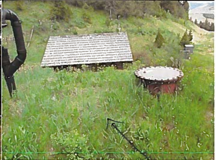
Mid Mountain tank 8000 gallon
