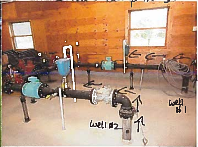
flow meter reading 43.0 gpm
