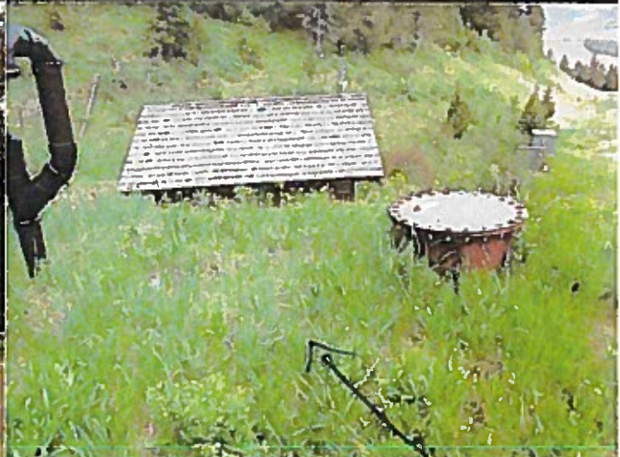
Midmountain tank 8000 gallon
