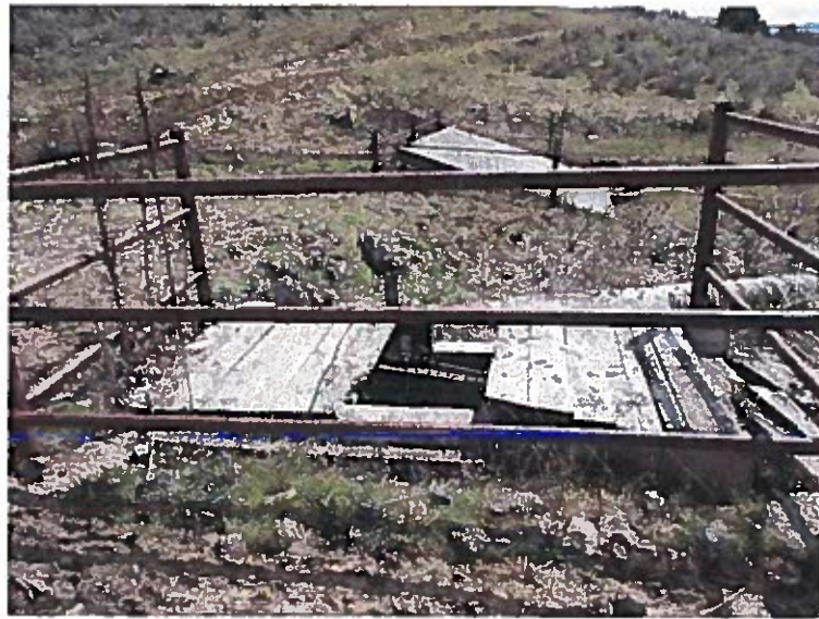
The headgates to the left release water into this weir.
