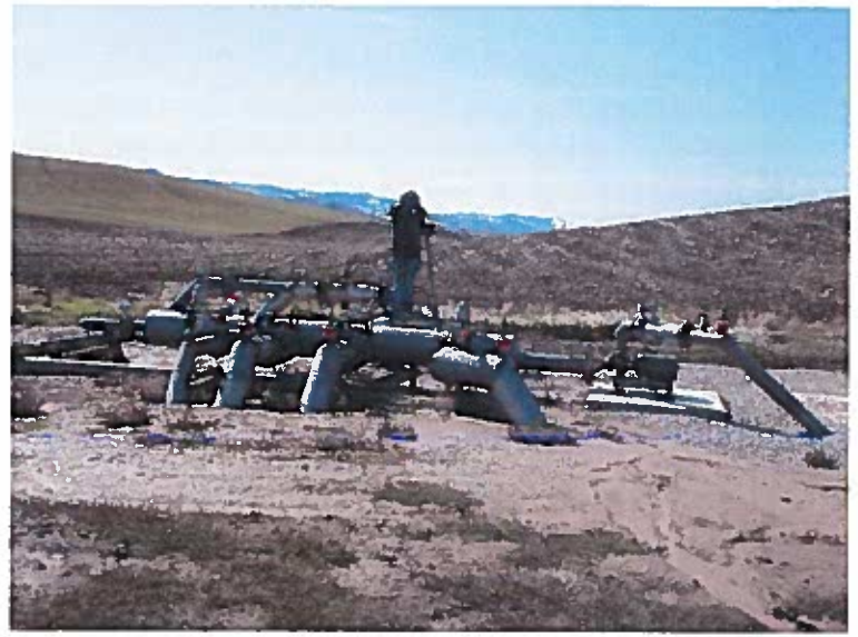
Irrigation system where water comes from weir down into the system and is then diverted out.
