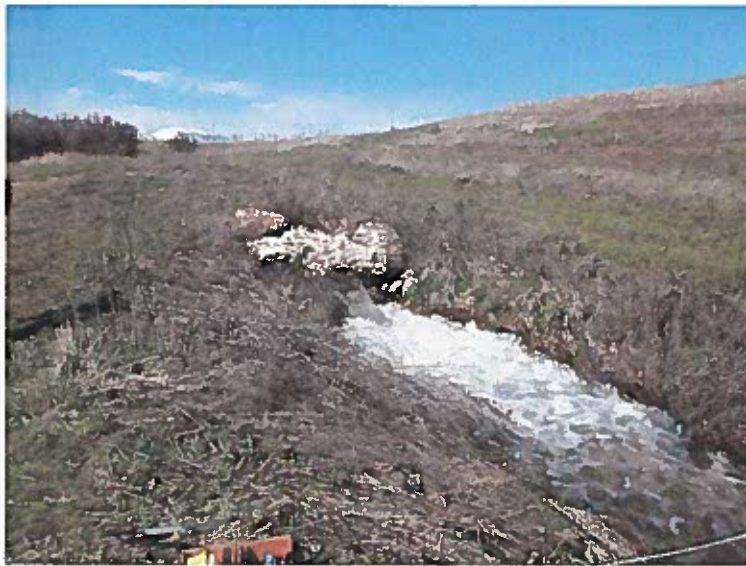
Discharge out of 12" CMP into fish propagation stream
