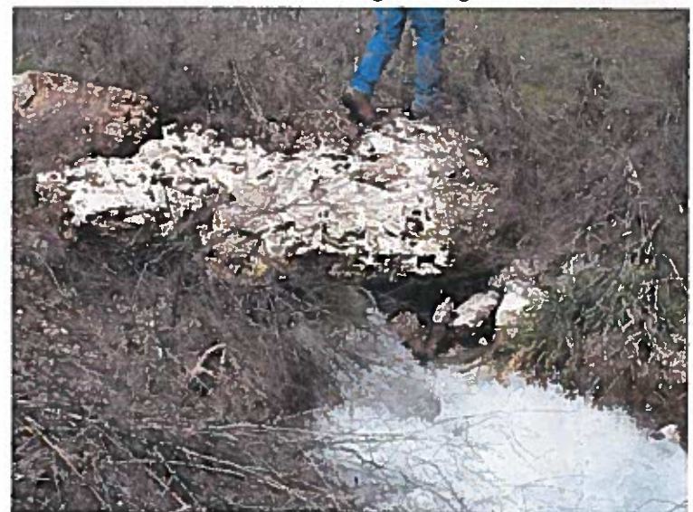
Close up of discharge out of 12" CMP
