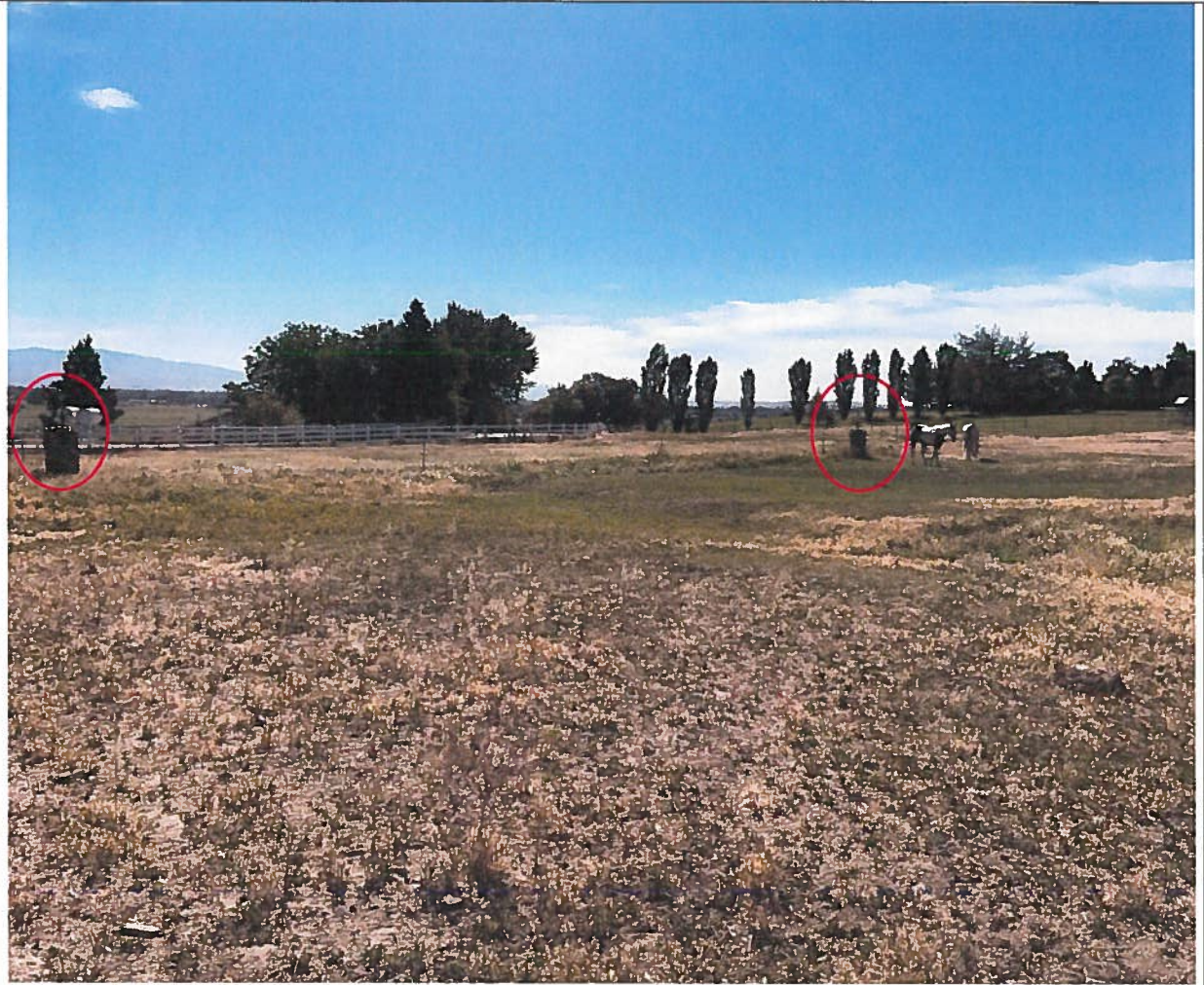
Photo 3: Place of use (POU) looking east. Two of the 15 big gun sprinklers visible and circled.
