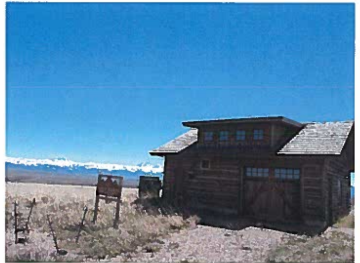
Booster pump station
