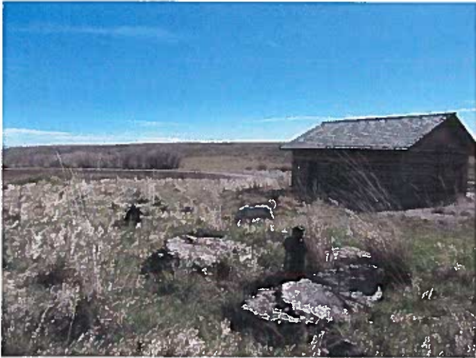
1 of 2 wells outside pump house
