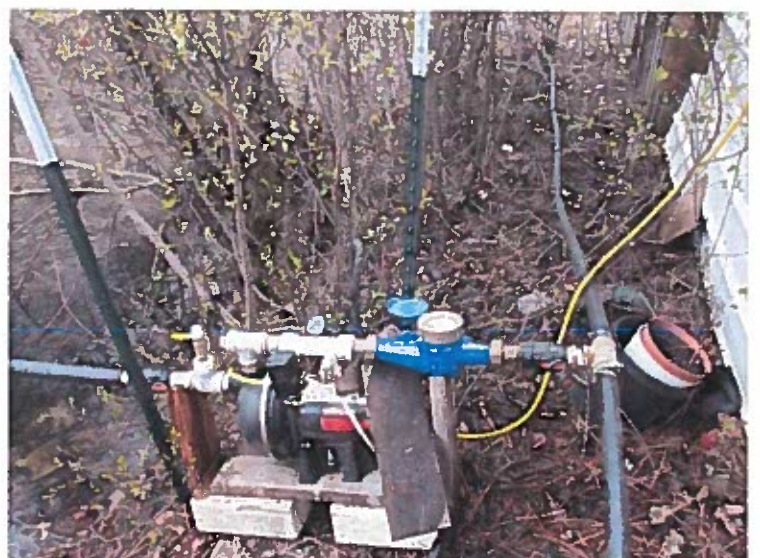
Close up of pump hooked up to the two pipes pumping the water to the east and west.
