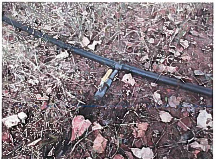
Ball valve for hose hook up. X5 on west side of the house.
