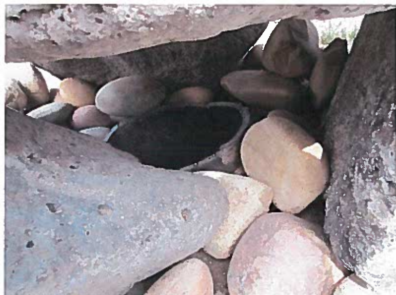
Pipe under rock where water is diverted into pond
