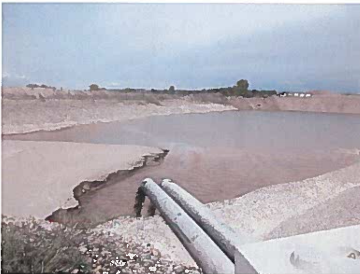
Water being discharged into the pond.
