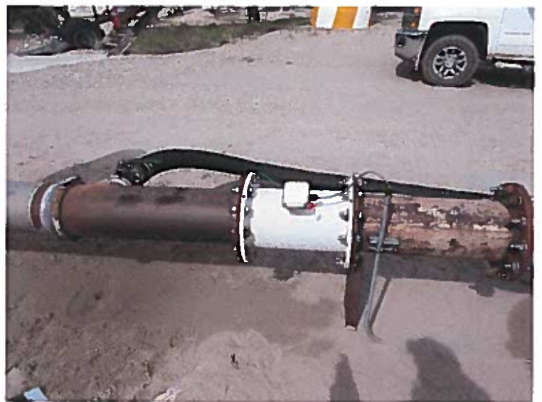
Picture of the system. Washing station on the top left. Installed Seametrics 2000-1000 flowmeter.
