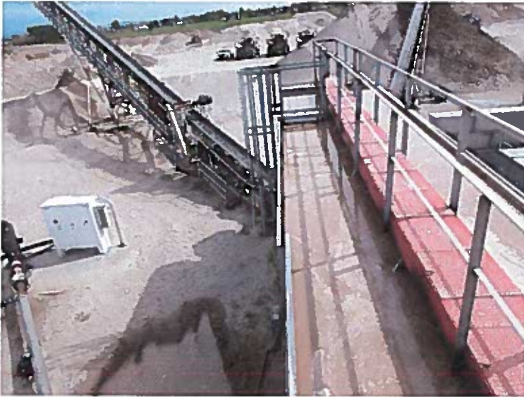
After gravel is washed it goes through a series of three settling tanks.
