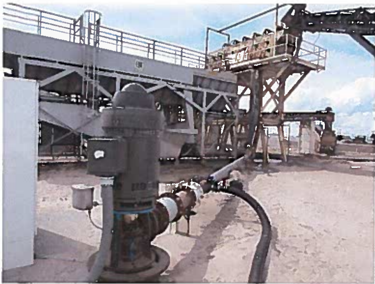
Picture of the system. Washing station on the top left. Installed Seametrics 2000-1000 flowmeter.
