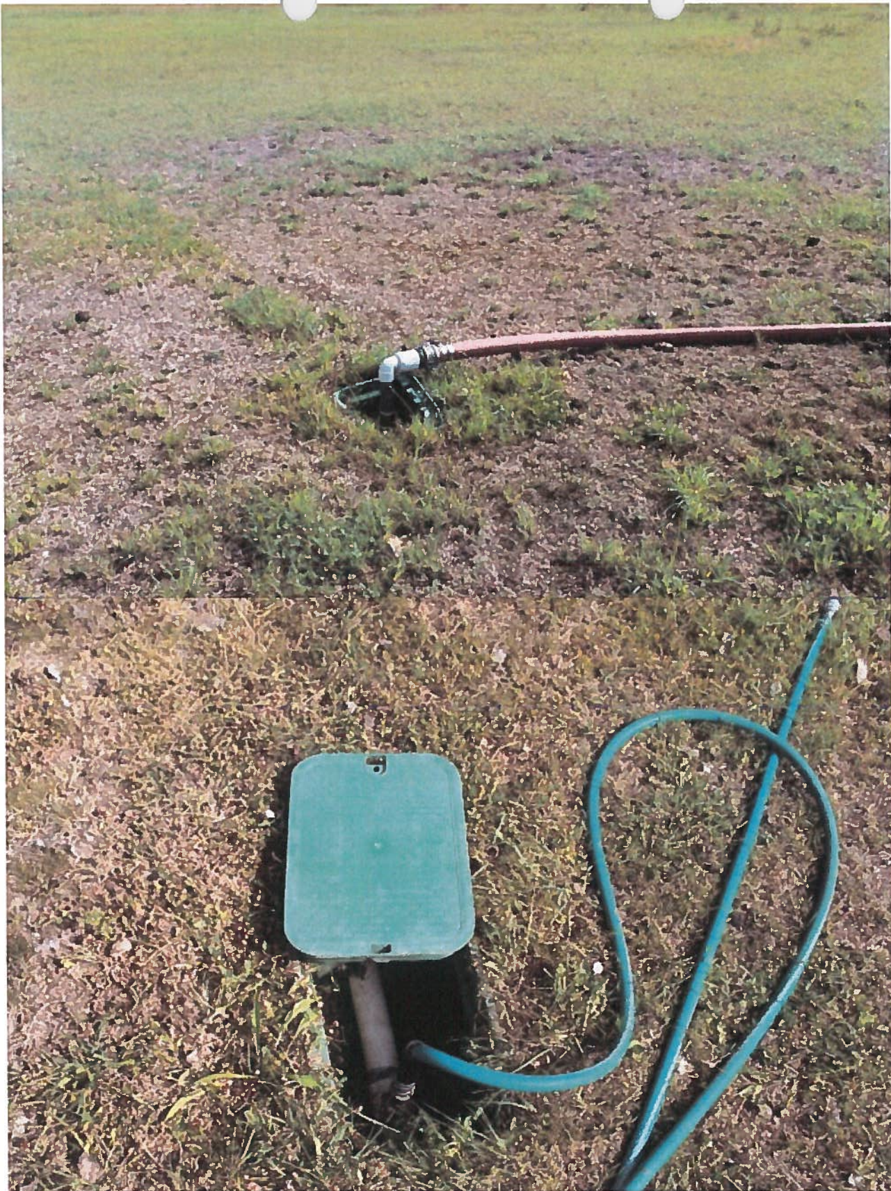
Diversion system WR# 65-23073
