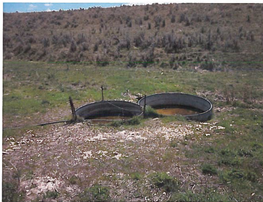
Figure 2: 12S28E15NENW . Elevation 4972 ft. Looking south to the overflow troughs fed by 1 ¼ inch poly pipe from sub-surface inlet control valve/overflow control valve
