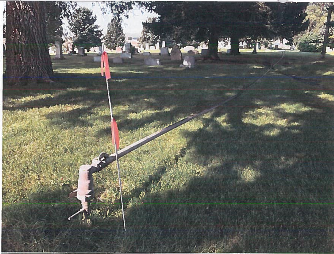
Riser with handline connected on north end of cemetery.
