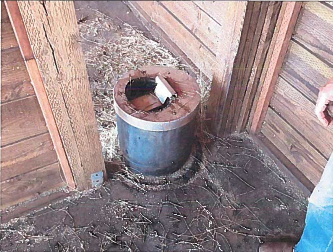
"Bar-Bar-A" non- electric trough. Horses or stock press flat lever and a water valve opens and fills the bucket.
